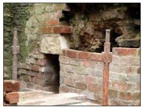
Fig 4 – Close-up of the capping stone on the top of the rebuilt flue on 11 February 2015.
