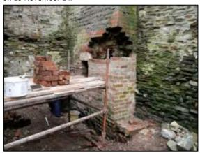
Fig 3 – Rebuild of the base of the chimney towards the end of 11 February 15 work party.
