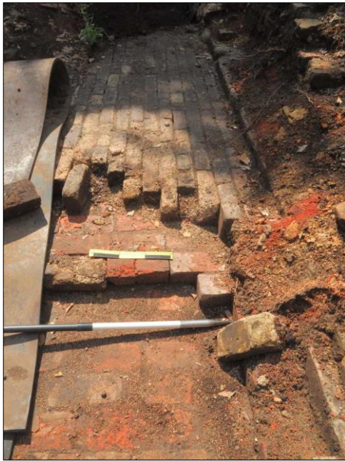
Photo 22 – Brick floor of the boiler setting furthest away from the Cornish Engine House. The brick courses in this setting run along the length of the setting (See comment on p.2). (1 m black/white ranging pole, 30 cm yellow/black scale)
