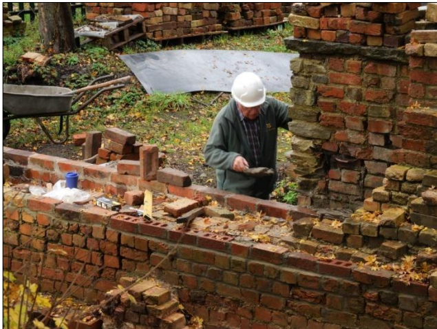
Photo 35 – Steve H works on rebuilding brickwork at the south-west end of the Egg-ended Boiler settings ...
