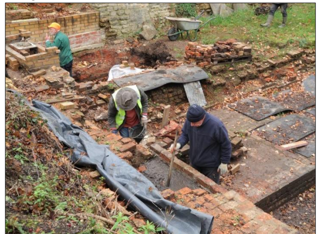
Photo 38 – In the foreground Hamish and Marek are backfilling with concrete, while in the background Ken can be seen building up a brick pillar.
