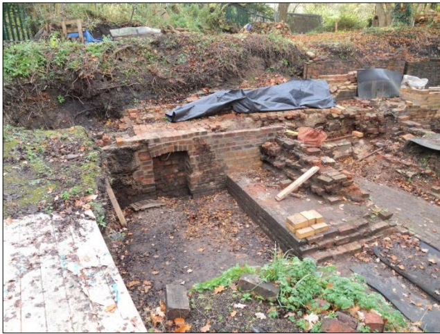
Photo 41 – The brickwork at the eastern end of the Lancashire Boiler settings during the rebuild (Note the rebuilt brick arch over the recess in the wall at the back left) ...
