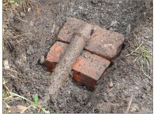
Photo 49 – The disconnected end of the pipe that runs from the chamber beside the vehicle gate to the New Pit yard. (see comments on p.2 )
