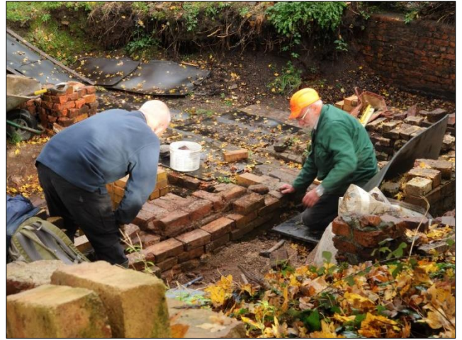
Photo 31 – Ken and Mick working on the conservation of the brickwork of Lancashire boiler settings nearest the Cornish Engine House in November ...
