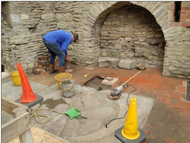
Photo 57 – Hamish working on repairs to the floor inside the Cornish Engine House (See comments on p.2 ). The red and the yellow traffic cones cover the two remaining engine holding down bolts ...
