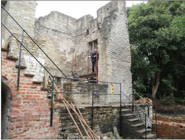
Photo 16 – Hamish and Marek dismantling the scaffolding tower inside the Cornish Engine House.
