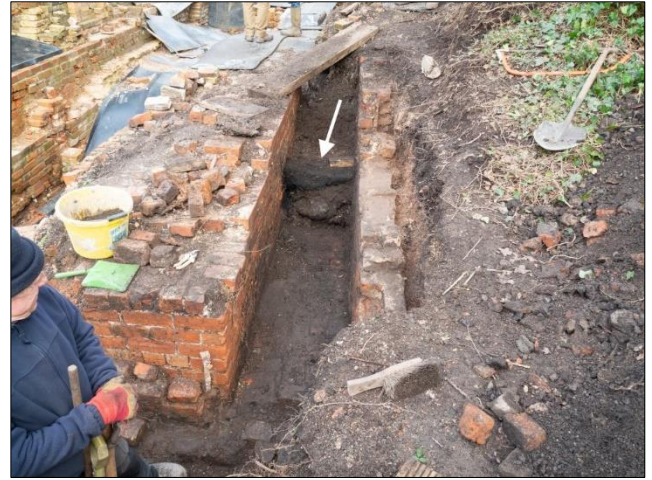
Photo 43 – A layer of dark material, possibly compacted coal dust, was found in the flue to the east of the Egg-ended Boiler settings. Here its position is marked by an arrow, while there is a close-up in the following photo ( 44 ).
