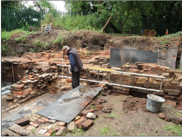
Photo 28 – Marek measuring the difference in heights between the two brick boiler bases in the New Boiler area. He is using as a reference point the top of a ladder, which was levelled with the aid of the yellow spirit level seen just behind him.
