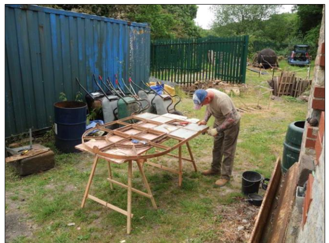
Photo 4 – John cleaning one of the cast iron window frames that will be fitted into the window openings of the Horizontal Engine House.
