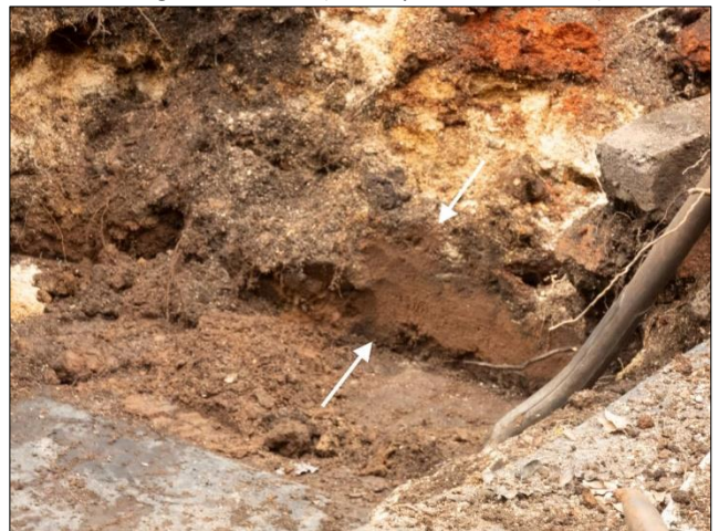
Photo 26 – A layer of a fine brown deposit, seen here marked by two arrows, has been found in various other locations within the boiler setting.
