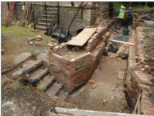
Photo 11 – A view along the Egg-ended Boiler settings as the scaffolding was being built outside the Cornish Engine House.
