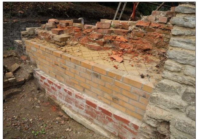
Photo 2 – The completed repairs to the bottom section of the wall seen in photo 26 of the previous newsletter (N° 36).
