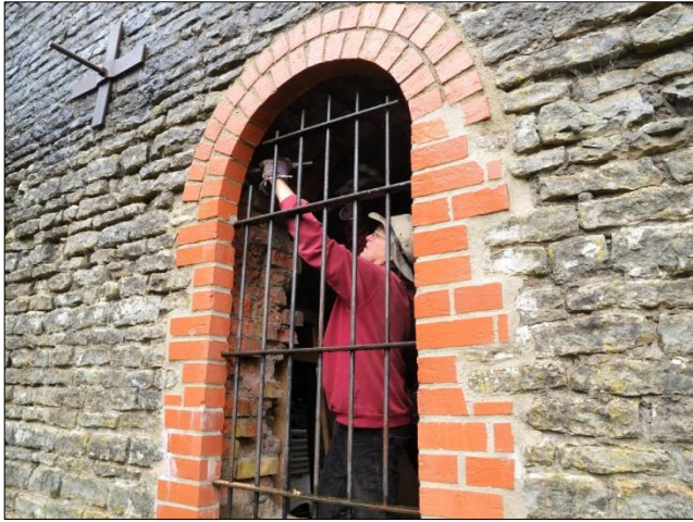
Photo 74 Pete W cuts a groove around the inside of one of the Horizontal Engine House windows, making it easier to fit the window frames.
