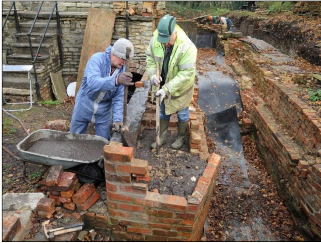
Photo 40 – Pete W and Steve H backfilling the newly built brickwork on the south-west end of the Egg-ended Boiler settings with concrete.
