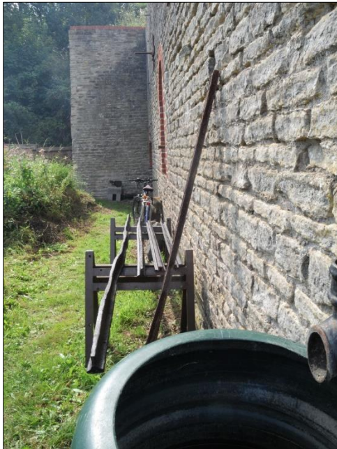
Photo 51 – The lengths of Dramway and Top Hat railway lines have been given a coating of WaxOil. The length of Dramway rail on the left is no longer straight. As the changes occur on the unsupported areas between the sleeper blocks, Hamish suggested that this was caused by a heavy load such as a loco.
