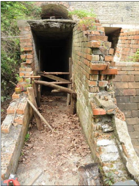
Photo 29 – View along the southern fan duct, looking towards the heapstead. Two Acrow props and a couple of home-made wooden props are being used to correct the inwards bow in the left hand wall.
