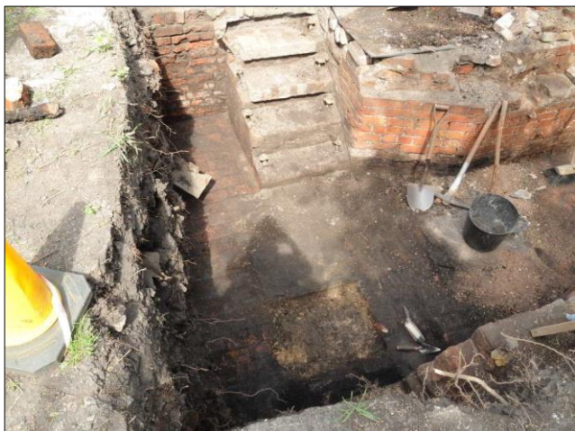
Photo 10 – The south-west end of the Egg-ended boiler settings at the end of April, with the new fence line just out of site on the left. The light coloured area at the centre of the bottom of the photo marks the spot where a stone slab had been removed ...
