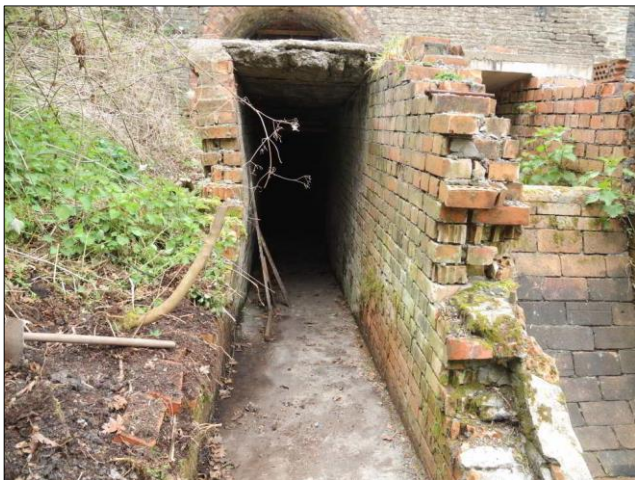
Photo 30 – For comparison this is a view along the same fan duct in April 2021. The 1" movement achieved so far is too small to be picked up from photographs.
