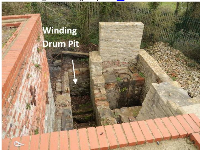
Photo 26 – The inside of the Vertical Engine House, showing the location of the winding drum pit.
