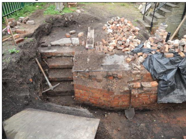
Photo 7 – Excavation in progress of the south-west end of the Egg-ended boiler at the end of March ...
