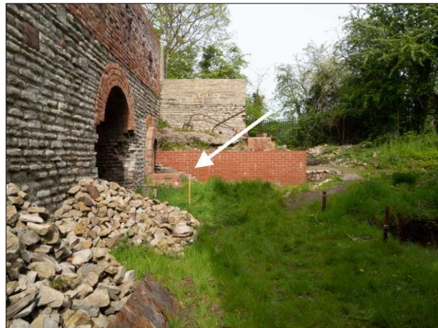
Photo 25 – The white arrow points to the stake marking the further point the radio sonde reached when pushed down the drain in the winding drum pit. The drain lies behind and to the left of the pale stone wall above the arrow, which is located just outside the right-hand edge of photo 26.
