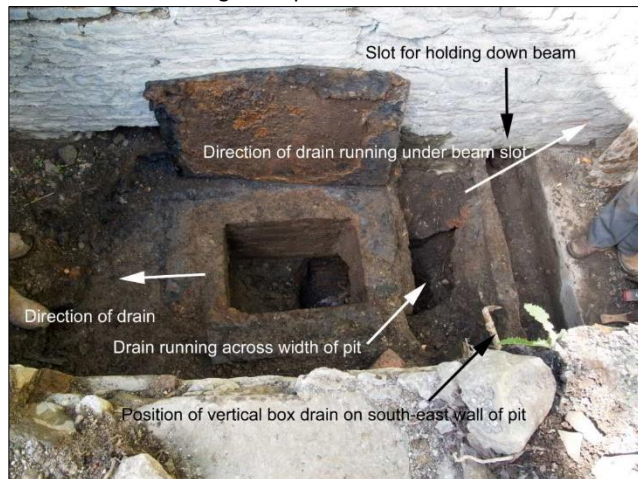
Photo 27 – The base of the winding drum pit in the Vertical Engine House in 2015. The drain under investigation on p.2 is the one on the left. (The one on the right runs in the direction of the Old Boiler House)
