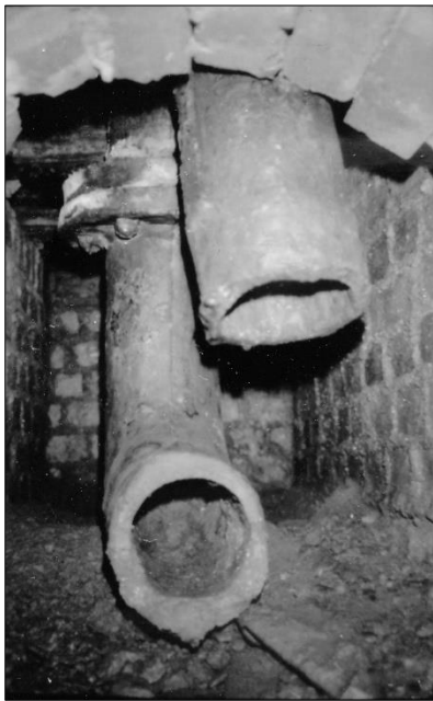
Photo 28 – 1986 photo of the water conduit, showing two pipes entering the conduit from above. (© B Turner, 1986)
