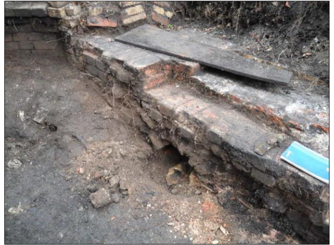
Photo 13 – The arched brick conduit in the south-east wall of the egg-ended boiler settings can be seen at the centre of the photo. The following photo ( 14 ) shows the inside of the conduit.
