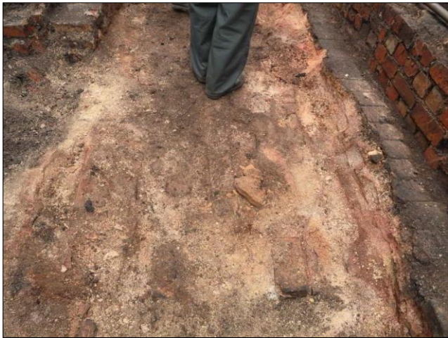
Photo 11 – The firebrick floor in this area has been affected by the heat of the flue gases.
