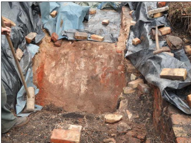
Photo 12 – The sloping section of the egg-ended boiler settings.
