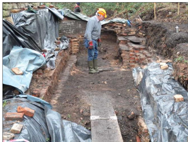
Photo 8 – Steve H inspecting progress. The plastic sheets are to protect the exposed brickwork from frosts.
