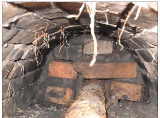
Photo 14 – Inside of the conduit seen in the previous photo ( 13 ). The end wall is a later addition as it is not keyed into the brickwork of the arched roof. The wall looks as if it was built around the metal pipe seen in the middle of the photo.
