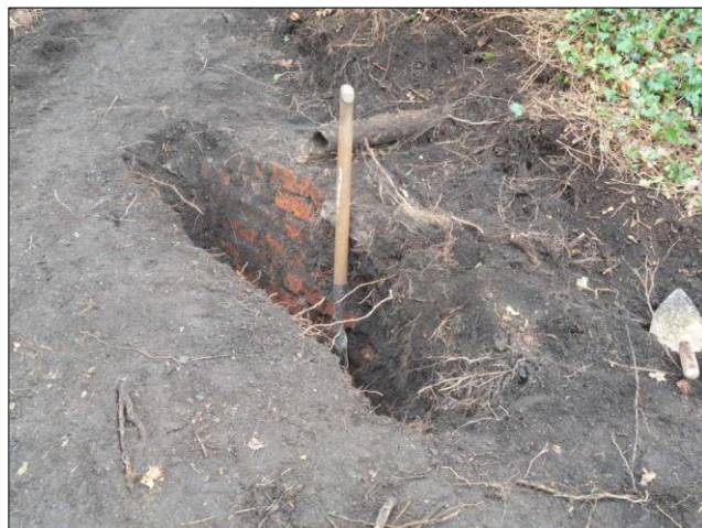
Photo 19 – This (~3" dia) metal pipe and brickwork appeared when the bank to the south-east of the egg-ended boiler settings was dug while relocating the adjacent path.
