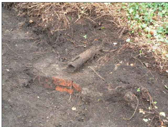
Photo 3 – This length of ~3" diameter pipe appeared when spoil was removed as part of the relocation of the path.
