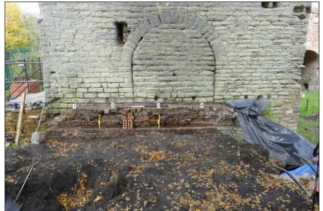
Photo 3 – The exposed brickwork at the base of the south-east wall of the Cornish Engine House. There is a close-up of the central section in photo 8 . The black/yellow scales are sitting on top of what may be the springing for a cover over the boiler. (1 m black/white horizontal pole, 30 cm black/yellow scales).
