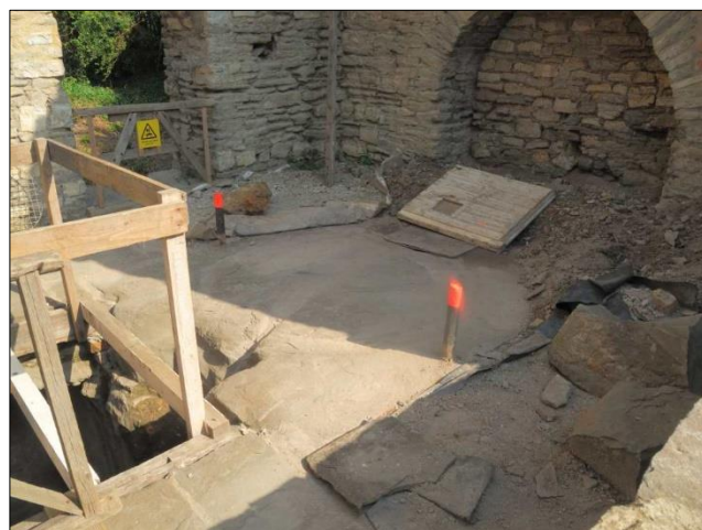
Photo 2 – The tops of the holding down bolts in the Cornish Engine House have been marked with pink paint as a hazard warning.
