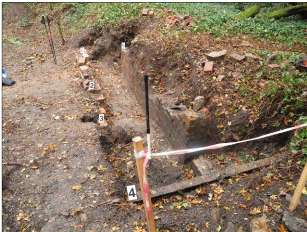
Photo 7 – Exposed brickwork along the line of the flue outside the new path from the New Boiler area. (1 m black/white vertical pole)
