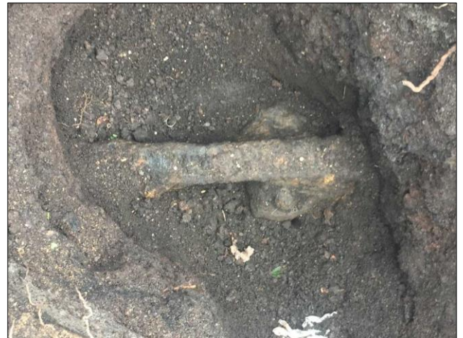
Photo 16 – ... the length of railway line he found, with a chair still attached. (© D Hore 2021)
