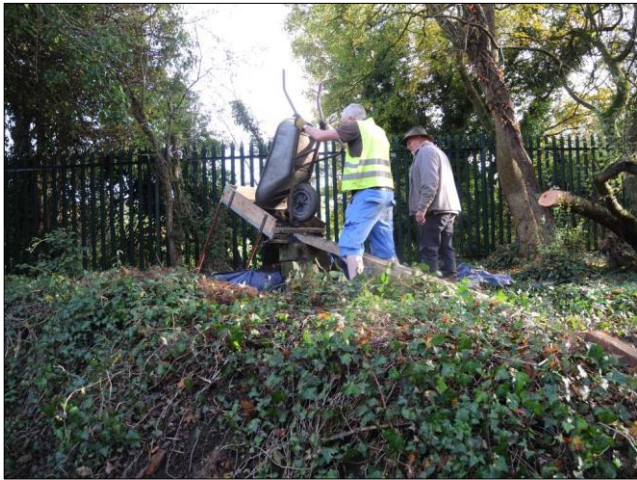
Photo 12 – Mark B dumps a barrowload of spoil on the sieve, while Hamish looks on. It is being used to sieve the ash-laden spoil lying on top of the foundations of the egg-ended boiler so that the spoil can be re-used at a later date.
