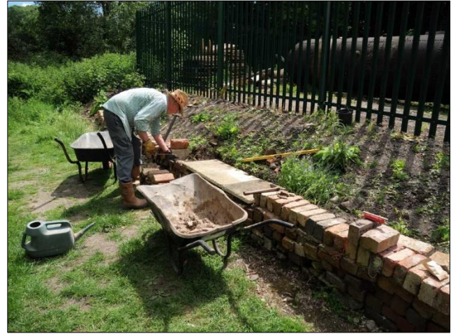
Photo 36 – Hamish laying bricks to form the retaining wall at the base of the slope near the egg-ended boiler. The flat area just above the nearest wheelbarrow is a seat that can be seen in the next photo ( 37 ).
