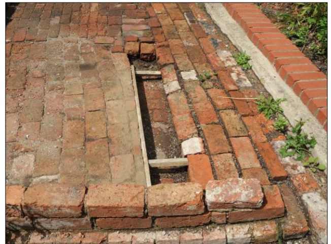
Photo 26 – Part of the building foundations on top of the Old Pit heapstead. The loose bricks to the left of the central strip of wood have now been mortared back in place. Photo 28 shows Mick working on this area.
