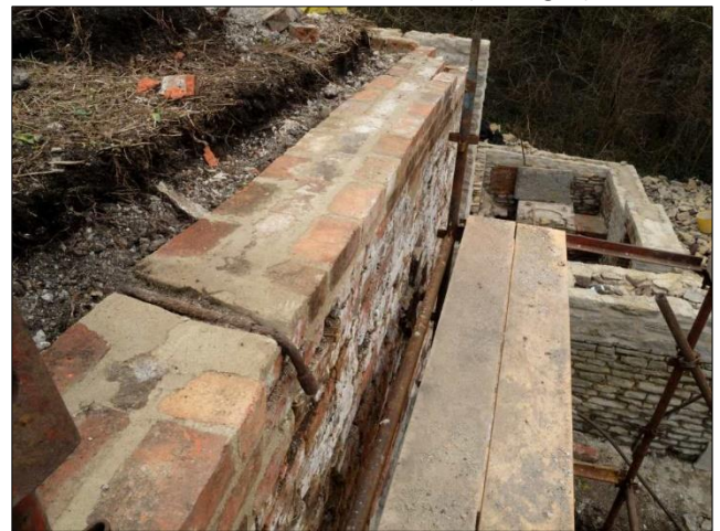
Photo 14 – Pipe discovered during the rebuild of the top of the south-east wall of the Old Pit heapstead in March 2016. (See comments on p. 2 )
