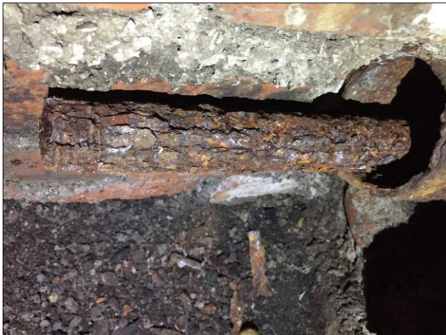
Photo 12 – ... which turns out to be an iron bar with what looks like a thread at the end. (© D Hore, 2021)
