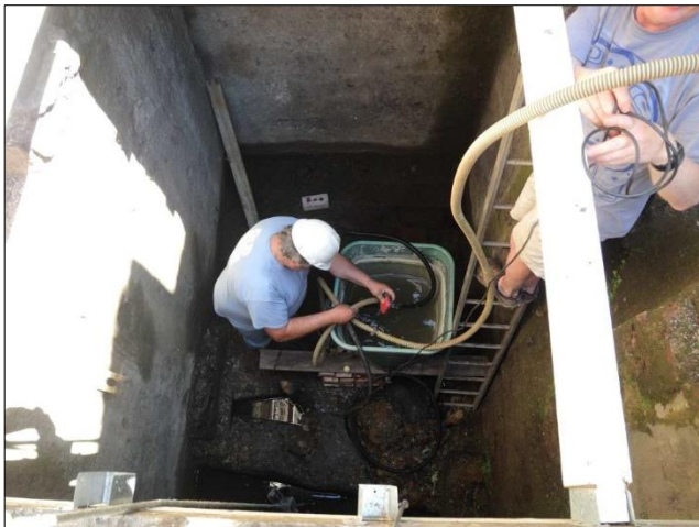
Photo 35 – Occasionally Mark B and others get to work in the condenser pit of the Cornish Engine House. Here Mark W is working at the bottom, pumping water out of the sump into a bin. The pump layout then had to be changed to pump the water out of the bin to the surface. Eventually the sludge in the bottom of the sump got the better of the pump, so it is back to the drawing board.
