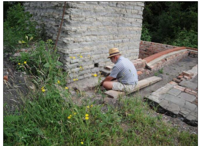
Photo 27 – Ken cutting out damaged brickwork at the base of the chimney.
