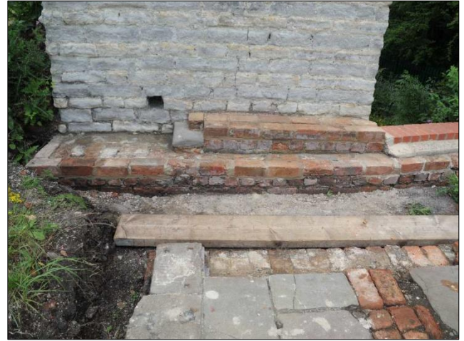
Photo 25 – Rebuilt section of wall running along the base of the south-east wall of the chimney.
