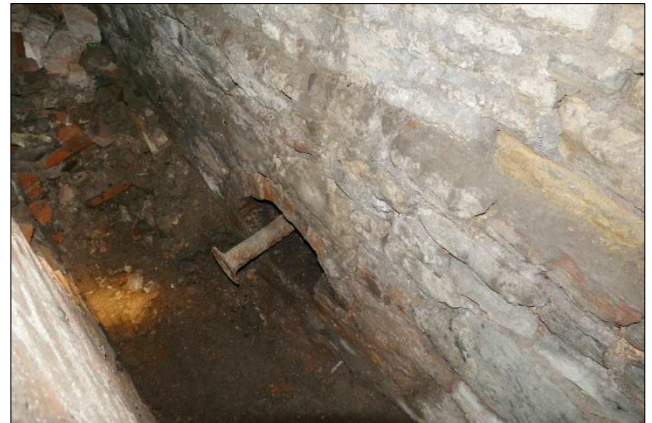
Photo 26 – ... and what is thought to be the other end enters the Horizontal Engine House undercroft through a brick archway at the base of the north-east wall. (November 2019)
