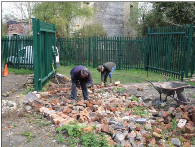
Photo 5 – Derek and Hamish building the hardcore entrance to the New Pit storage area.
