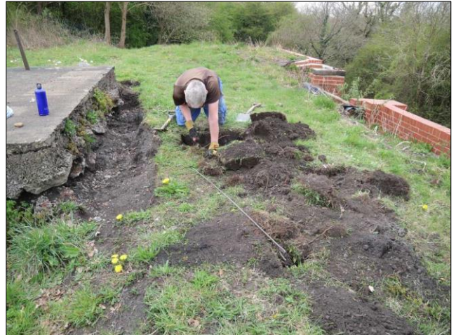
Photo 12 – Mark working on test pits on the north-west side of the New Pit shaft capping.
