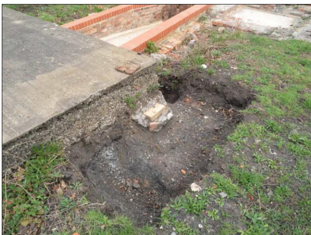
Photo 11 – Exploratory pits at the eastern corner of the New Pit shaft capping, with the winding ramp at the top of the picture. (See comments on p.2)
