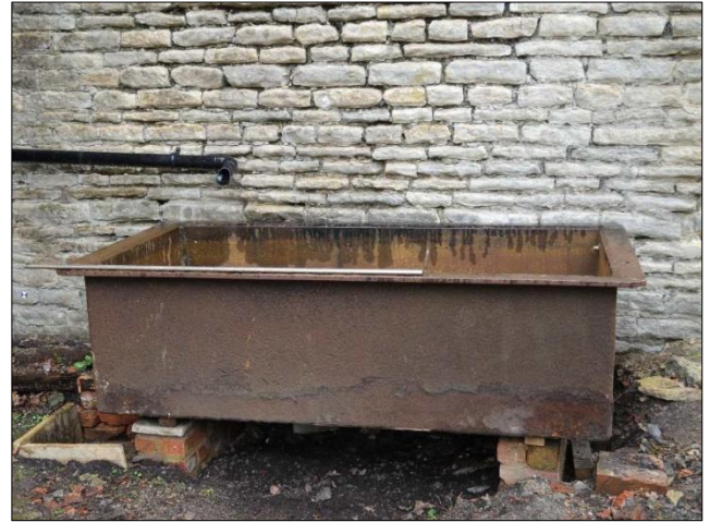
Photo 24 – The tank in place. Rainwater collecting in the winding ramp on top of the heapstead now drains into the tank through the black pipe.
