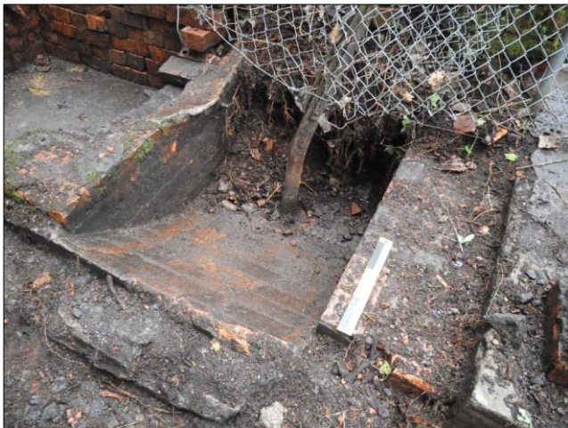
Photo 7 – This 2016 photo shows the fence pole inserted into the brick base of the fan housing. (30 cm scale at the inside edge of the right-hand brick plinth)
