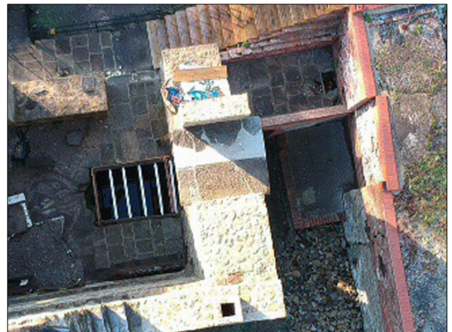
Photo 10 – This enlargement of the bob wall shows how the fragments of one of the pivot stones have been set into the top of the bob wall - See comments on p.2. (© Tarquin Powell 2020)
