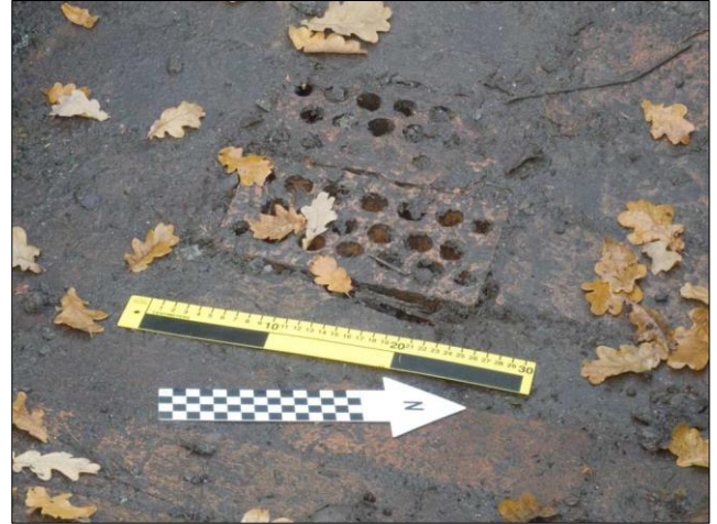
Photo 8 – The perforated bricks act as a drain at the bottom of the fan housing. The fence pole seen in photo 7 had been inserted at the corner nearest the head of the north arrow. (30 cm yellow/black scale)
