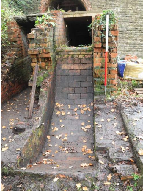
Photo 6 – A view of the fan housing from a position outside the line of the old boundary fence. The two perforated bricks that form the drain are located towards the bottom of the photo. (1m red/white ranging pole)
