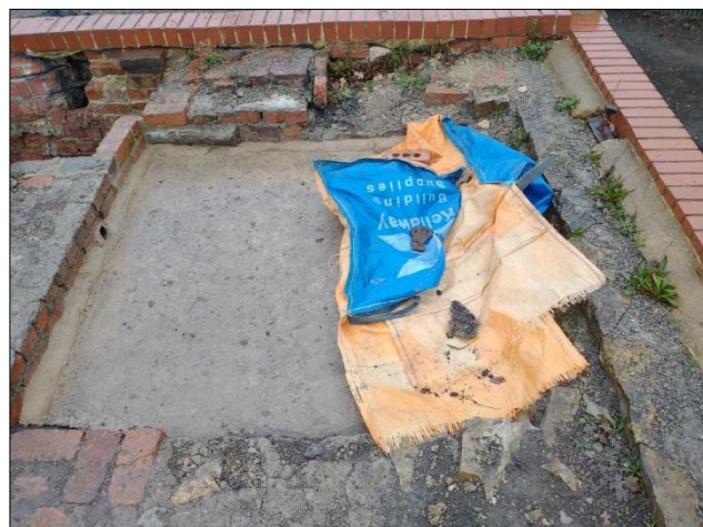
Photo 4 – This area to the south-east of the winding ramp has had the concrete floor and water-proof membrane sealed to the wall with a cement flaunch. (© Mark Bonson, 2020)
