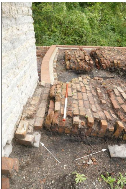
Photo 24 – View of the collapsed walls on the north-western side, with Area C in the foreground and Area A in the background. The two stones marked by arrows in the foreground have holes drilled into them (see comment on p.3). (1 m red/white ranging pole)
