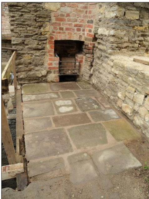
Photo 3 – The northern corner of the Cornish Engine House with its new flagstone floor. The edge of the condenser pit is on the left-hand side of the photo ...
