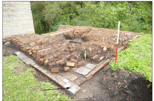
Photo 22 – Overall view of the brick structures at the north-east end of the Old Pit heapstead. The stone in the foreground marked with an arrow has holes drilled into it (see comment on p.3). (1 m red/white ranging poles and 30 cm yellow/black scale)
