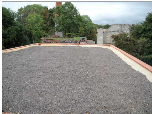
Photo 5 – View of the top of the Horizontal Engine House from the New Pit heapstead. The white area running around below the bricks on top of the walls is the new flaunching (see comments on p.2 ).
