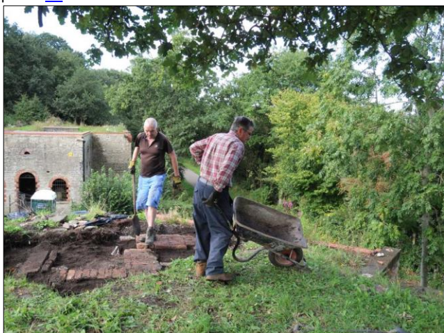
Photo 21 – Mark and Derek start to backfill the area around the structures at the south-west end of the Old Pit heapstead. They first covered the brickwork with a layer of sieved spoil, then a waterproof membrane followed by a final layer of spoil.
