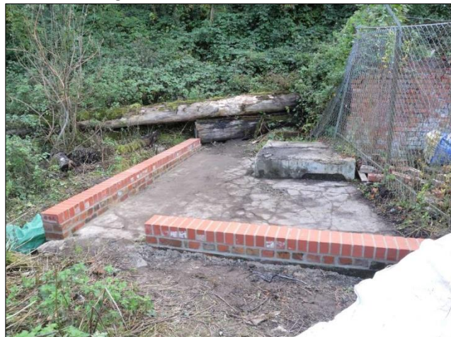
Photo 7 – The replacement low wall built along the edge of the fan house using reclaimed bricks capped with a row of modern bricks.
