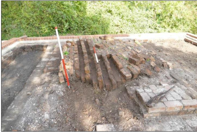
Photo 29 – Area A has been partly dismantled, showing the arrangement of headers and footers. (1 m red/white ranging poles)
