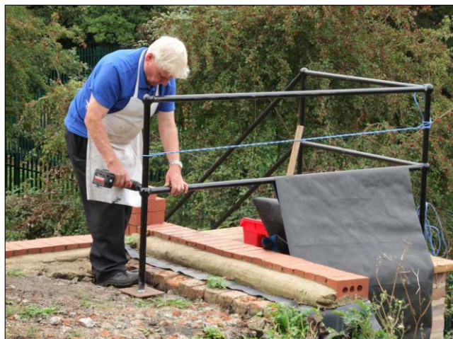
Photo 36 – Jeff completing the safety railings for the steps at the south-western end of the Old Pit heapstead.
