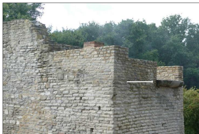
Photo 2 – View of the Cornish Engine House from the top of the Old Pit heapstead, with the northern corner of the building in the foreground. The arrow marks the position of the pivot stones.
