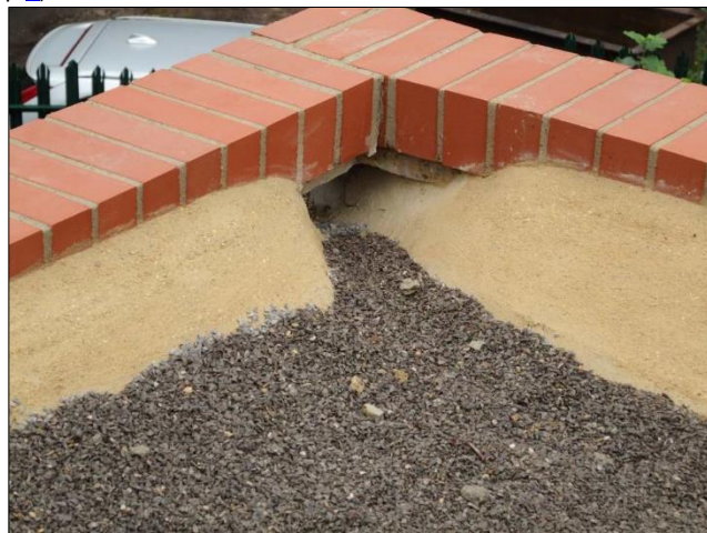
Photo 6 – Close-up of the flaunching at the drain in the northern corner of the engine house.
