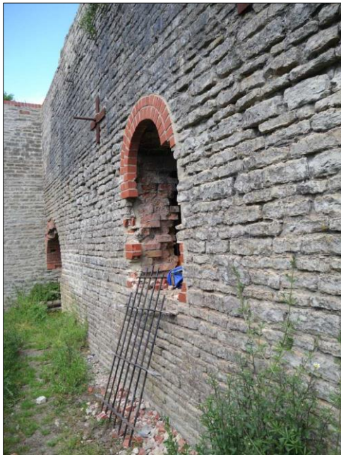
Photo 9 – The extent of the damage to the brickwork surrounding the window in the south-east wall of the Horizontal Engine House in May 2019.
