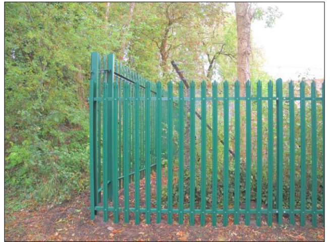
Photo 11 – ... and the same spot at the next work party. The 8 ft high palisades have been added and the 7 ft high section in the foreground runs along the edge of the cycle path.
