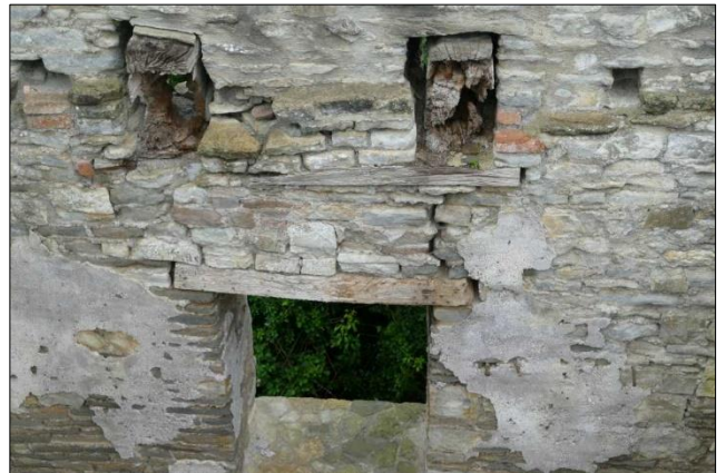
Photo 46 – ... and a close-up of the area around the remains of the wooden beams. There are smaller sockets for subsidiary beams on either side of the main sockets.
