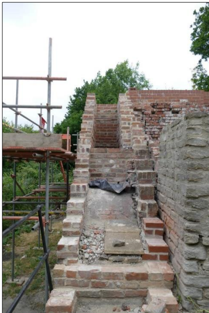
Photo 1 – View of the rebuilt brickwork at the south-west end of the Old Pit heapstead. Photos 5 and 6 in the previous newsletter (Nº 27) show the original layout and the vandalised state respectively from the same viewpoint.
