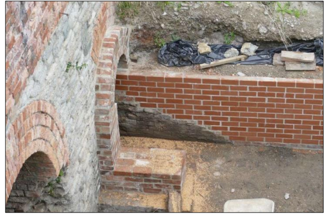
Photo 15 – This view of the brick arch was taken from the scaffolding around the bob wall. It clearly shows the join between the original and new brickwork, and how the bricks of the arch now extend beyond the face of the heapstead wall.
