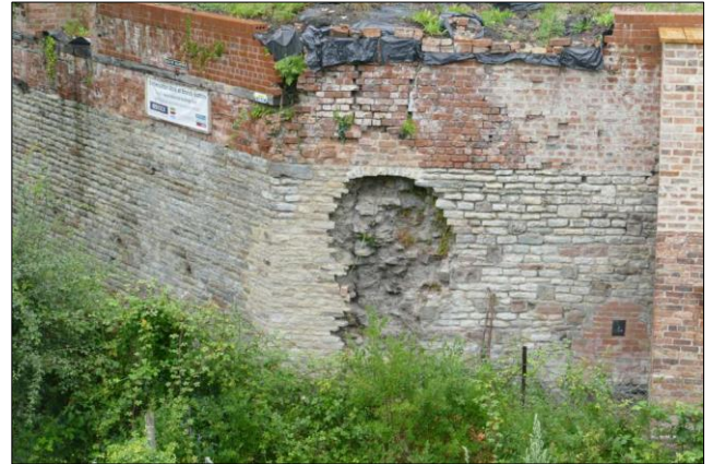
Photo 9 – Hamish built a masonry arch that connected the two parts of the stone facing. He also rebuilt some of the brickwork immediately above it, improving the stability of the rest of the wall.
