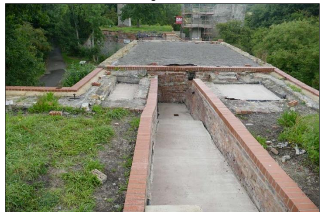
Photo 22 – The winding ramp of the New Pit heapstead after a waterproof membrane covered by concrete was laid in July 2020. (See comments on p.2)
