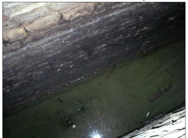
Photo 28 – Another view of the south-eastern wall of the chamber, looking downwards to the water level. This photo was taken during dry weather, and the dark area on the wall shows the range of water levels. The bright area at the bottom of the photo is the reflection of the flash.
