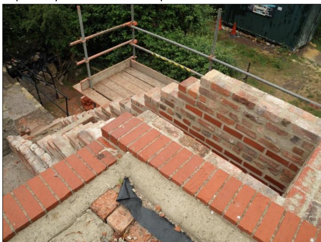
Photo 2 – A view of the same area as the previous photo, but this time taken from the top of the heapstead. This view makes it easier to see the layout of the reinstated steps ...
