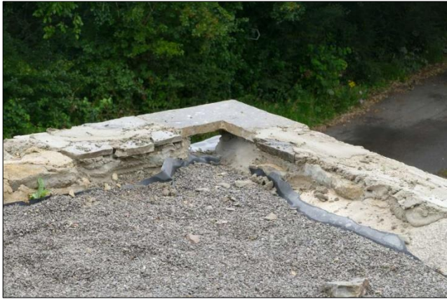
Photo 24 – A stone bridge has been laid as a support for the coping brick course over the drainage channel in the northern corner of the Horizontal Engine House roof ...
