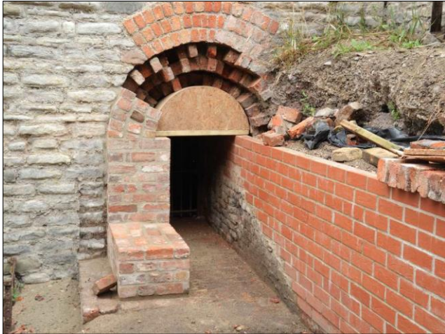
Photo 13 – The brick arch at the end of the East Flue during the rebuild ...
