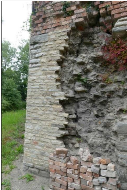
Photo 8 – The masons completed the rebuild of the western corner of the Old Pit heapstead. Photo 13 in the previous newsletter, N° 27, shows the same area during the rebuild.
