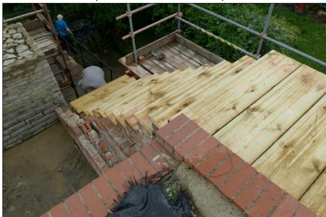
Photo 3 – ... and with the wooden treads in place.
