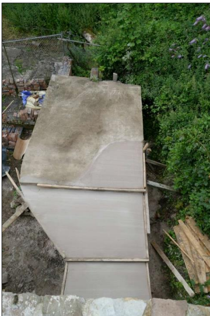
Photo 20 – The newly cast roof of the fan ducts, seen here from the top of the New Pit heapstead, now extends from the fan housing, situated at the top of the photo, to the wall of the shaft. The camera angle gives the impression that there is a considerable difference in height between the top and bottom sections, though photo 21 shows that this is not the case.
