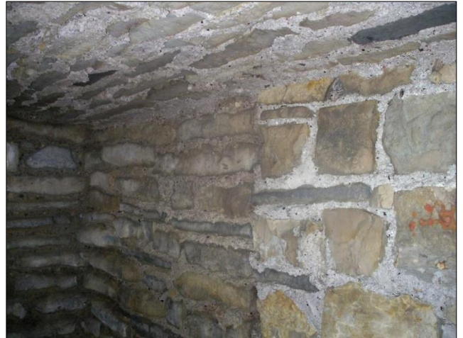
Photo 27 – View of the south-eastern wall of the chamber at the south-eastern end of the Cornish Engine House. The vertical break in the stone courses does not run the full height of the wall.
