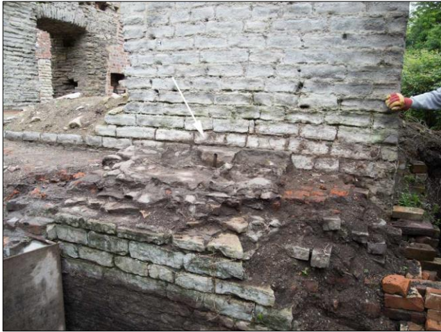
Photo 18 – The platform outside the south-west wall of the Cornish Engine House in July 2017. The arrow points to a stone that had a hole drilled upwards – see comments on p.2.
