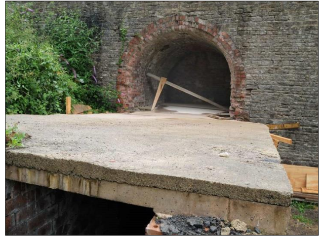
Photo 21 – View of the new roof from the fan end of the ducts with the shuttering still in place. This angle shows that the roof is at almost the same level throughout.
