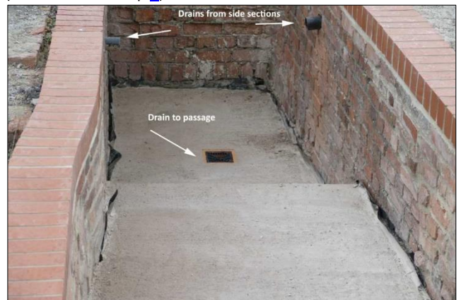
Photo 23 – View of the Horizontal Engine House end of the winding ramp, showing the arrangement of the drains.
