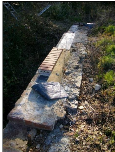
Photo 8 – ...The same wall showing that almost all of the capping has been demolished by the vandals. (© K Kemp 2020)
