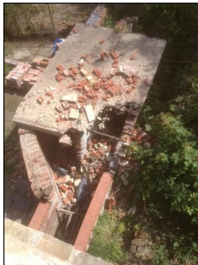
Photo 12 – There was more damage to the roof of the fan ducts during the second wave of vandalism. (© H Orr-Ewing 2020)
