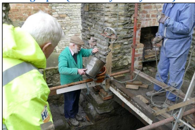
Photo 1 – Jeff watches Ken pouring some muddy sludge, dredged from the bottom of the condenser pit, into a funnel connected by a pipe to the sump in the Old Pit alcove.
