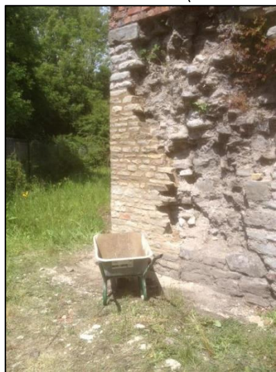
Photo 13 – Repairs underway to the stone facing of the western corner of the Old Pit heapstead. (© H Orr-Ewing 2020)
