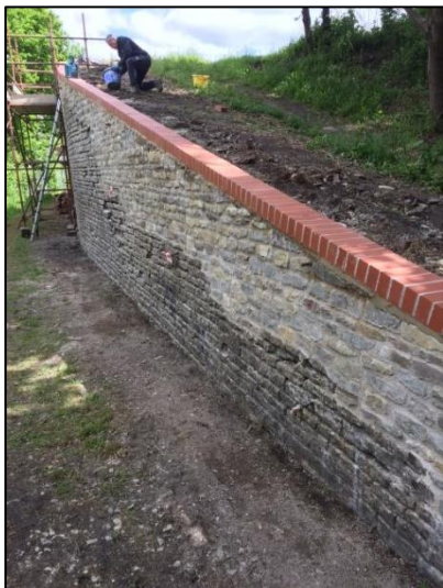
Photo 9 – The recently rebuilt face of the cycle path side of the New Pit heapstead ramp. (© H Orr-Ewing 2020)
