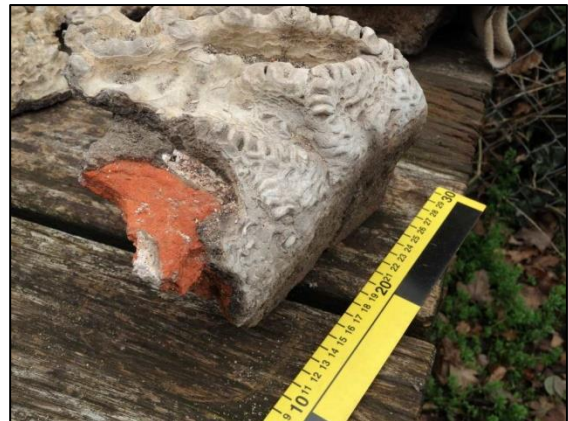
Photo 12 – This piece of the edge of the brick arch (BB 090219-2) was found in the top level of the spoil. It has been inverted for photography, and the rough lime scale deposit on the 'top' would actually have been on the underside of the arch. (30 cm scale)
