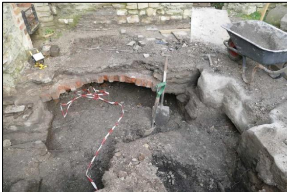
Photo 10 – The exposed edge of the brick arch on the north-east side of the building. The wheel barrow on the right is sitting on the engine bed.
