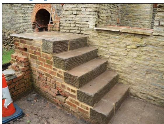
Photo 1 – Steps outside entrance to Vertical Engine House in January 2019. There is still some repointing to be completed on the brickwork at the bottom of the base.
