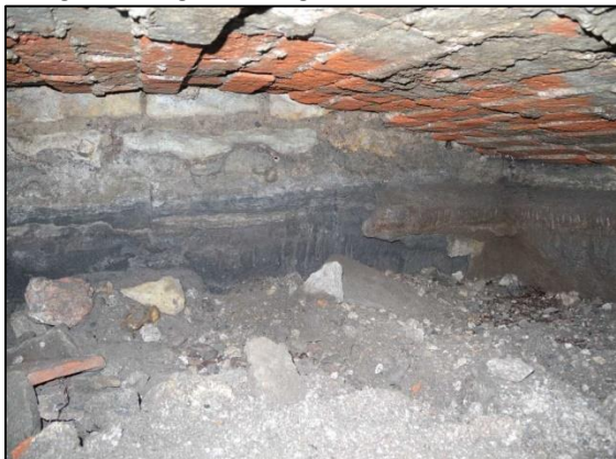
Photo 11 – View looking north-eastwards into the cavity seen in the previous photo. Note the shallowness of the arch.
