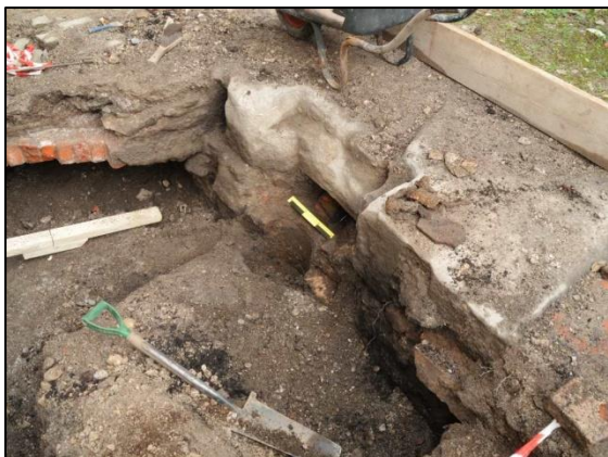
Photo 15 – Close-up of the engine bed area of the excavations in the Cornish Engine House. The bed is in the top right of the photo. Below it, and just to the left of the 30 cm yellow/black scale, is a semi-circular groove cut into the engine bed foundations.
