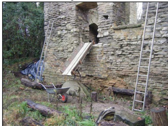
Photo 8 – A chute has been made to direct the spoil removed from the inside of the Cornish Engine House into a waiting wheel barrow ... (© M Taylor 2019)
