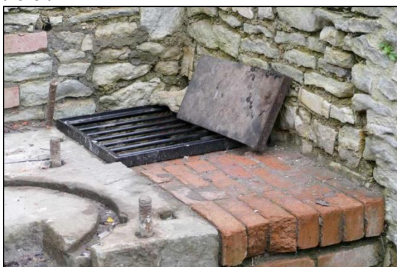
Photo 4 – The opening to the south-east of the engine bed of the Vertical Engine House has been closed with a metal grate – one of the many examples of Jeff's metal working skills to be found on site.
