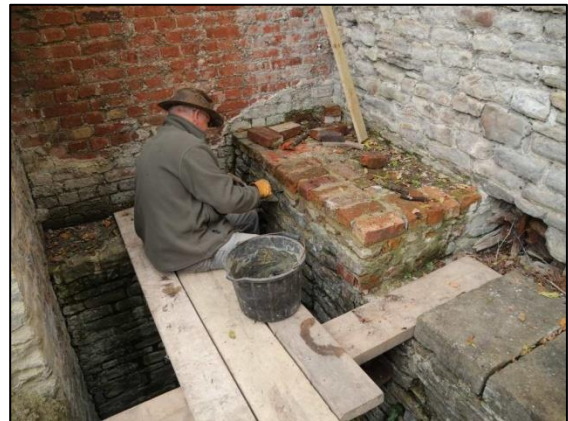
Photo 5 – Missing bricks have been replaced on the platform in the western corner of the Vertical Engine House.
