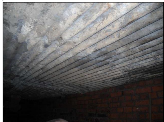
Photo 30 – The underside of the false floor of the Horizontal Engine House, taken at the south-western end of the central bay of the undercroft.
