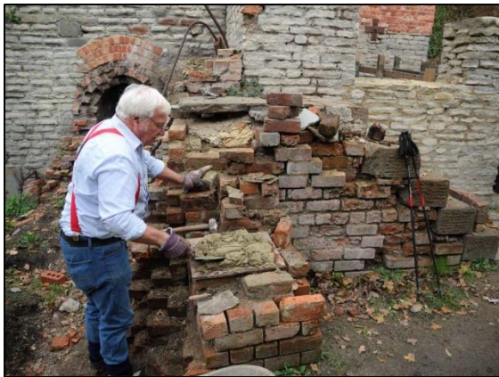
Photo 7 – Rebuilding in progress of the brickwork under the steps outside the entrance to the Vertical Engine House.
