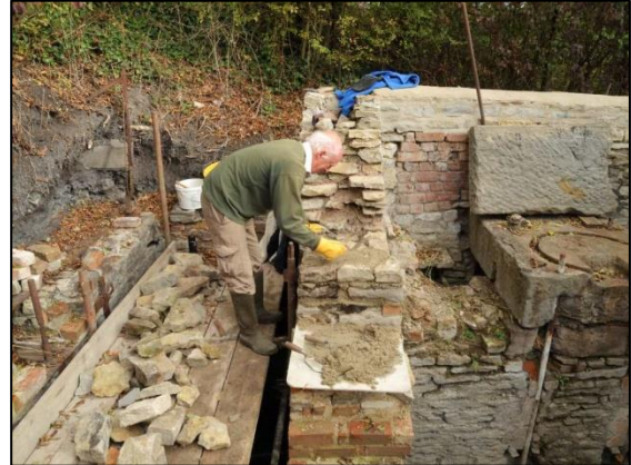
Photo 4 – Rebuilding the wall between the winding drum pit (on the left) and the engine bed in the Vertical Engine House.
