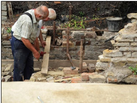
Photo 3 – ... During the rebuild, the edge of the rebuilt beam slot in the south-eastern wall was aligned with that of the existing slot in the north-western wall.
