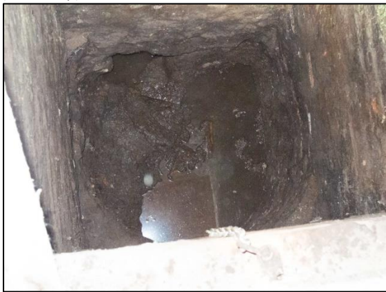
Photo 21 – The recently deepened bottom of the well in the Old Pit alcove. The conduit seen towards the top left of the photo goes under the heapstead.
