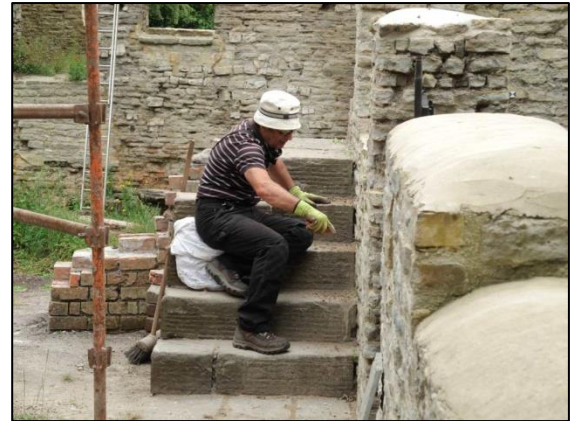
Photo 10 – Preparing the area seen in photo 7 for repointing.
