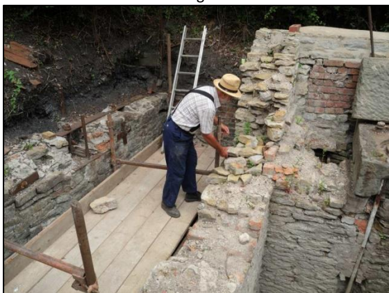
Photo 2 – Getting ready to rebuild the wall between the winding drum pit and the engine bay in the vertical Engine House.
