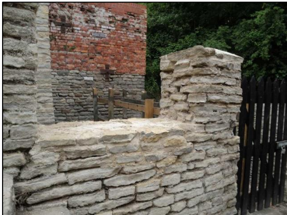
Photo 9 – ... and the almost finished result – a stone sill has still to be fabricated and laid. The area has been repointed after the photo was taken.
