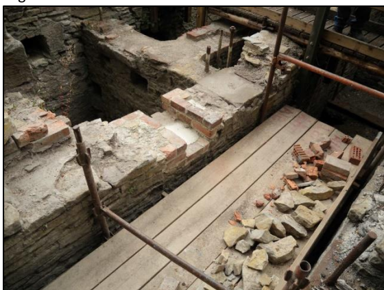
Photo 3 – The wall between the winding drum pit and the engine bay after the channel between the two had been rebuilt.
