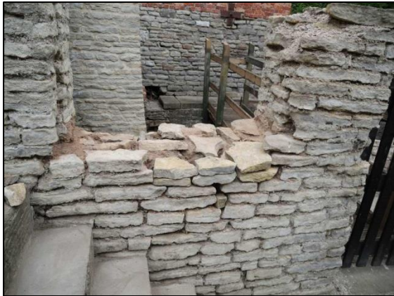
Photo 7 – ...after the loose mortar was cleared away ready for rebuilding ...
