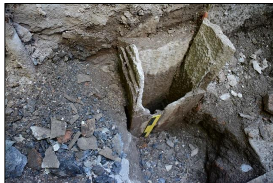
Photo 4 – Photo of scale deposited around the walls of a riser in the winding drum pit, Vertical Engine House, taken in 2015 as the spoil was being removed.
