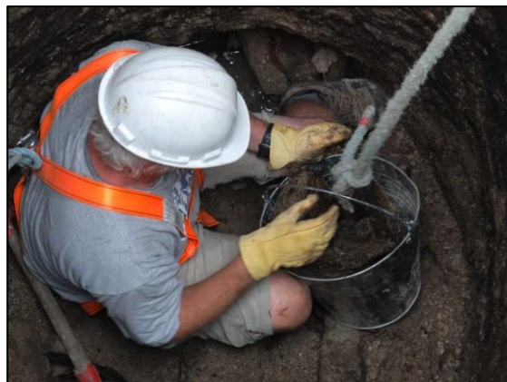
Photo 17 – Excavating spoil from the bottom of the shaft outside the entrance to the Vertical Engine House ...
