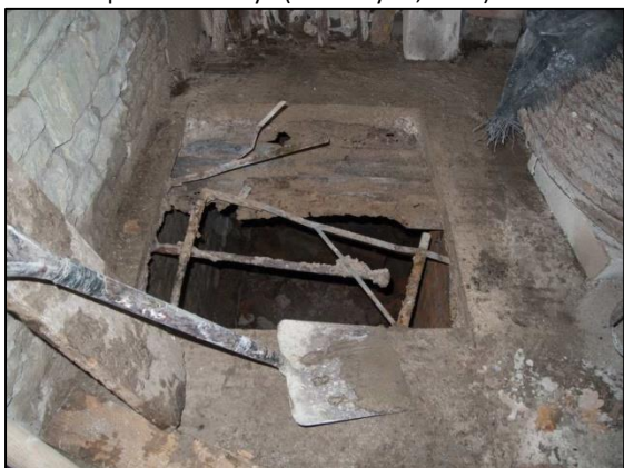
Photo 10 – The hole in the process of being punched through the concrete floor of the Horizontal Engine House to create a new entrance to the undercroft.
