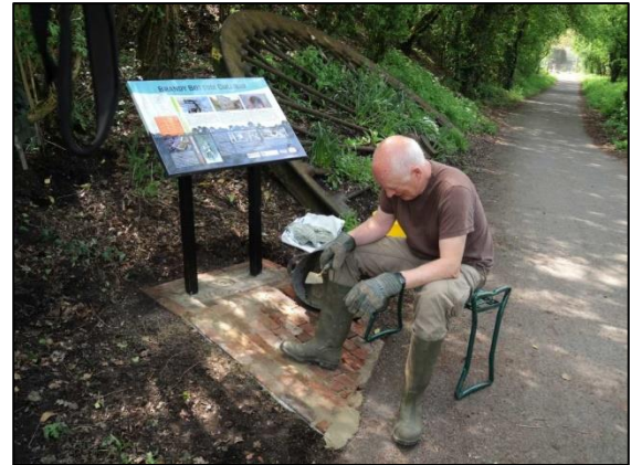
Photo 18 – ... grouting the gaps in the path ...
