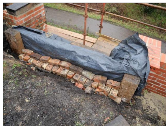
Photo 2 – Old bricks laid as drainage at the bottom of the trench along the back of the southern New Pit tippler slot. The trench has now been backfilled.
