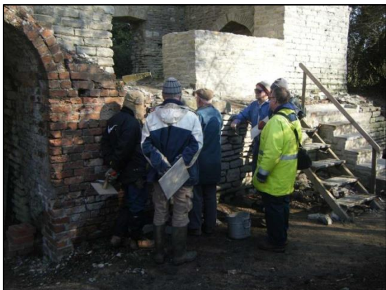
Photo 9 – ... and the class watches as they are shown how to repoint masonry. (© M Taylor, 2018)
