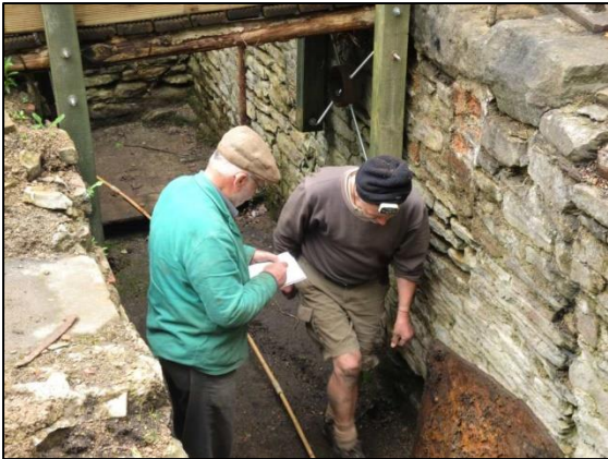
Photo 15 – Rodding the drains at the bottom of the winding pit in the Vertical Engine House, in an attempt to find out where they go.
