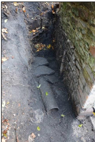
Photo 7 – A metal pipe, covered by stone slabs at the far end, outside the entrance to the Old Boiler House.
