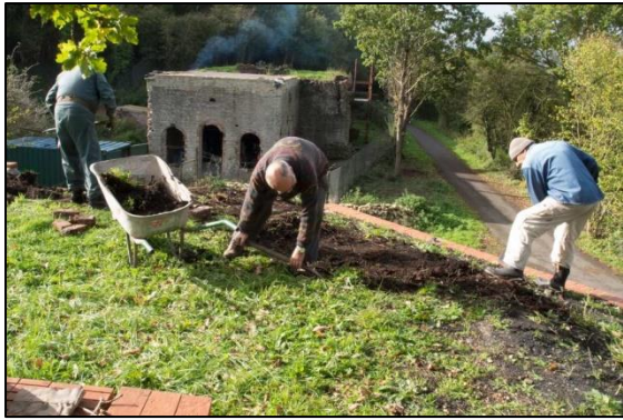
Photo 13 – The area at the south-western of end of the Old Pit heapstead being covered up with a layer of spoil on top of a plastic sheet.
