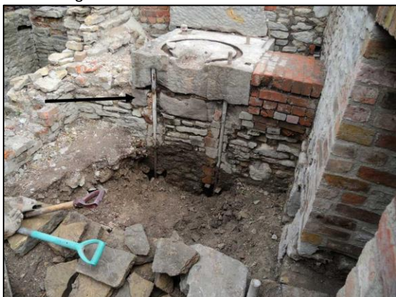
Photo 2 – Photo of the engine bed of the Vertical Engine House in 2012. The arrow points to what may be the bed of an earlier engine.
