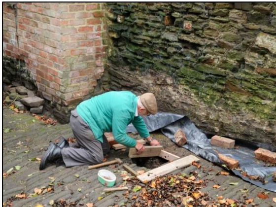
Photo 14 – Building a support frame to stop the sides of a hole in the floor of the Old Boiler House from collapsing inwards.
