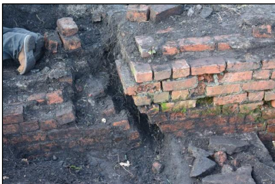
Photo 2 – Crack in the north-west wall of the New Pit winding ramp.
