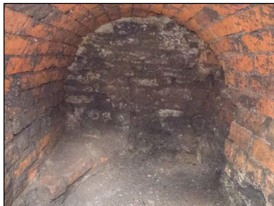
Photo 22 – The inside of the alcove. This has a brick ledge on the left, and is connected to the platform above by a hole on the top right of the arch.
