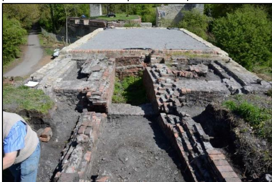
Photo 21 – The partially uncovered winding ramp of the New Pit heapstead. The gap between the walls narrows towards the Horizontal Engine House.
