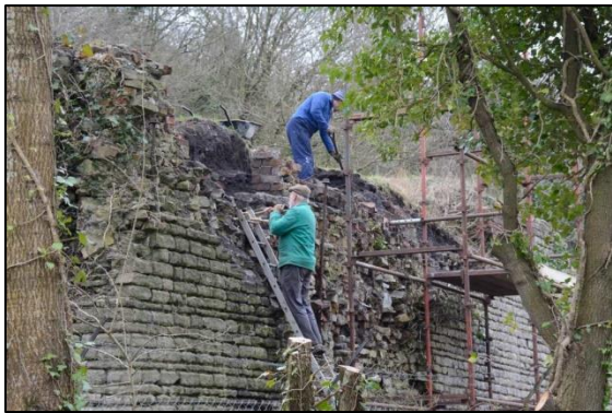
Photo 14 – The length and direction of the drain pipe in the north-west wall of the New Pit heapstead is probed, while spoil clearance continues above.
