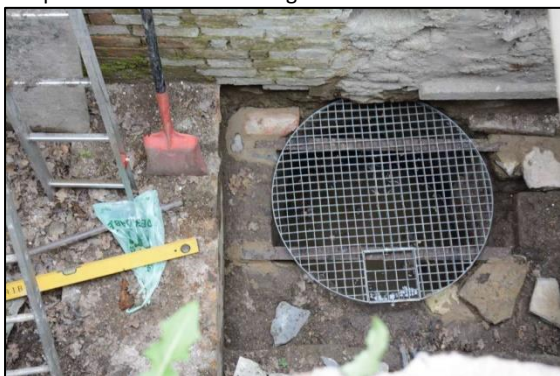
Photo 27 – ... and the cover is temporarily put in place to check the fit.
