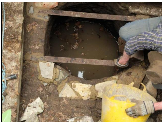
Photo 26 – Building the supporting framework for the sump cover in the Vertical Engine House ...
