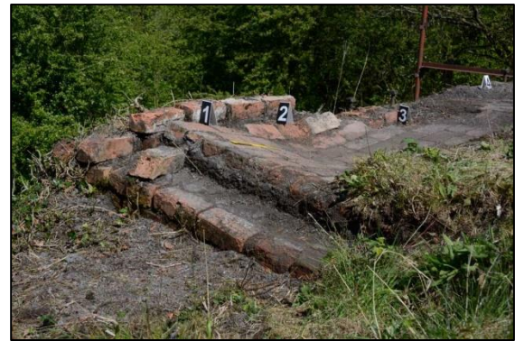
Photo 17 – The same corner as in photo 16, but from a different angle that shows the subsidence in the area around the '2' more clearly.
