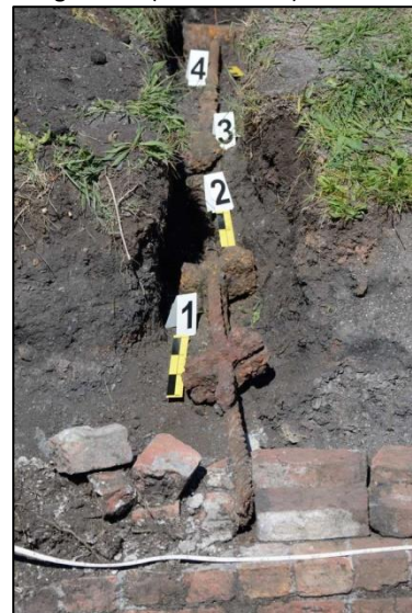
Photo 19 – The wire rope and anchorage point in-situ to the north-west of the winding ramp, New Pit heapstead. (30 cm scales)
