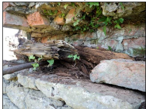
Photo 12 – The inside of the left hand end of the slot, containing a fragment of the original wooden beam.
