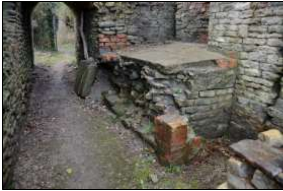
Photo 13 – This February 2014 photo shows the state of disrepair of the masonry walls below the capping of the Pumping Shaft.
