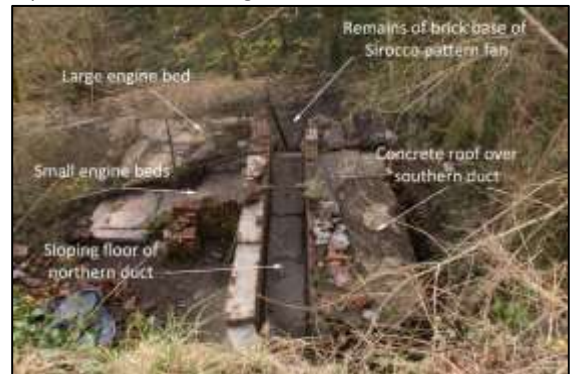
Photo 24 – View of the fan ducts from the top of the New Pit heapstead. Taken at the end of February, it shows the new brickwork on the top of the northern wall and the position of the fan housing. A close-up of the small engine beds was shown in the photo on page 7 of Newsletter N° 10.
