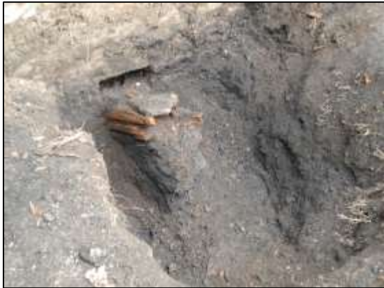
Photo 51 – Remains of timber bracing beam at base of southern wall of Old Pit heapstead.
