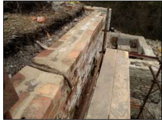
Photo 53 – The top of the south-eastern wall of the Old Pit heapstead squared off ready for capping. This photo also shows the position of the conduit seen in the following photo.
