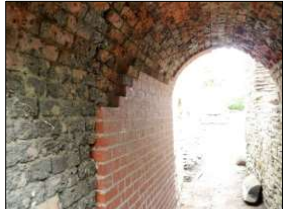
Photo 17 – Inside of the Pumping Shaft passage, showing the rebuilt section of wall on the left.
