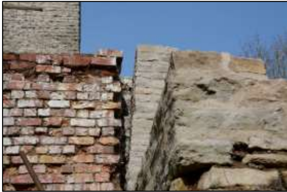
Photo 1 – Close-up of the top of the finished buttress in the Vertical Engine House, showing the gap between the original wall of the engine house and the brick top of the heapstead.
