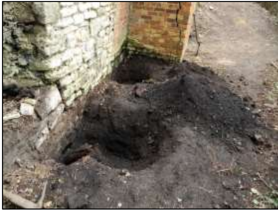
Photo 50 – The holes show where bracing beams had been positioned, thought to support the bridge seen in the 1881 map between the Old Pit heapstead and the Horizontal Engine House. A close-up of the timber in the nearest hole can be seen in the next photo. This area has been covered up again.
