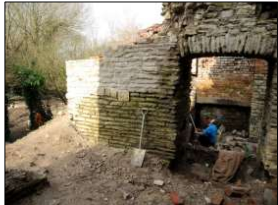
Photo 11 – ... and in March 2016 after the building of the supporting buttress on the left of the arch.
