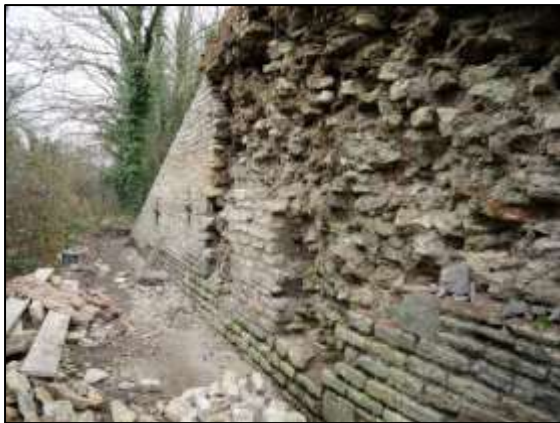
Photo 25 – A pillar is being built upwards to support the brick top of the north-western wall of the Old Pit heapstead.
