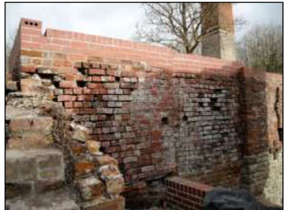
Photo 36 – ... and the same corner in April after the top of the wall was rebuilt and capped.
