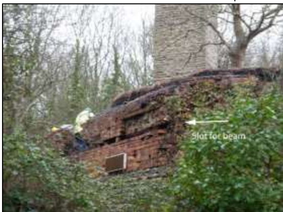
Photo 39 – The southern end of the north-western wall of the Old Pit heapstead, showing the gap in the brickwork where the wooden beams had been.
