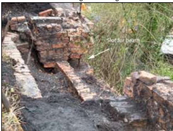
Photo 38 – The dilapidated state of the brickwork around the southern tippler slot before reconstruction started. The end of a slot which should have held a wooden beam can be seen in the centre of the picture.
