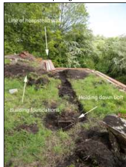
Photo 55 – North-eastern corner of Old Pit heapstead, showing the position of the building foundations (photo 56) and holding down bolt mentioned on page 5.
