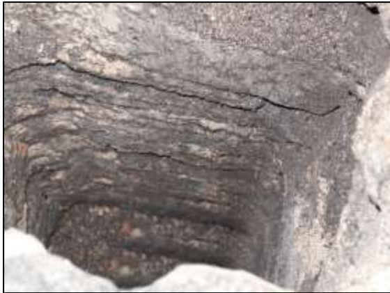
Photo 19 – The inside of the stone lined shaft located in the platform above the Pumping Shaft.
