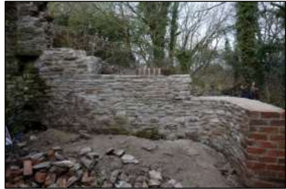
Photo 6 – The northern corner of the Old Boiler House in March after rebuilding.
