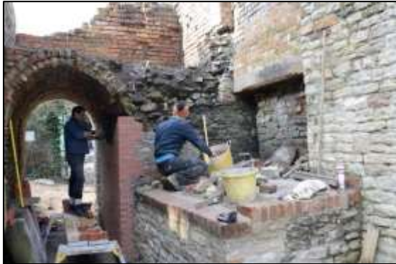
Photo 14 – Masons at work rebuilding the inside of the Pumping Shaft passage, and the wall above the shaft capping.
