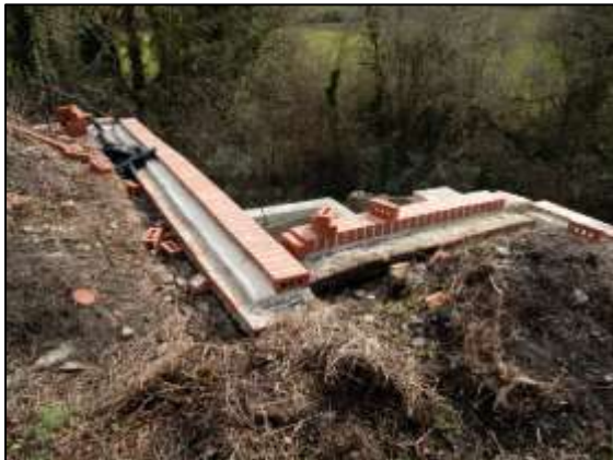
Photo 33 – Capping in place along the edge of the Old Pit heapstead wall above the Vertical Engine House.
