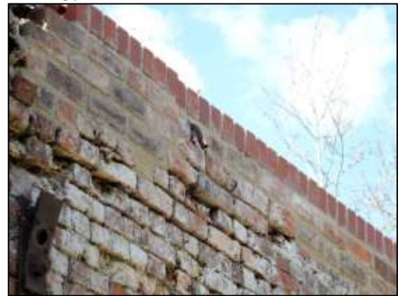
Photo 54 – The conduit poking out of the rebuilt wall.
