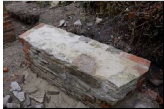
Photo 4 – The same length of wall after rebuilding in March but before capping.
