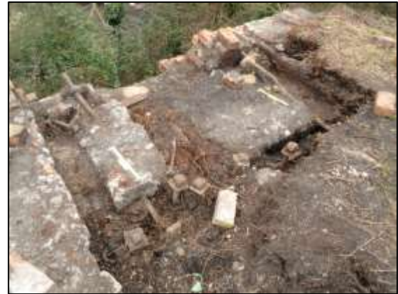
Photo 47 – Two wire ropes were uncovered at the south-west end of the Old Pit heapstead, clamped to the wall. The photo shows their anchorage points after the area was cleared of spoil, with the remains of a wooden beam running along the line of bolts. The anchorages can be seen in close-up in the next two photos. (30 cm scales)
