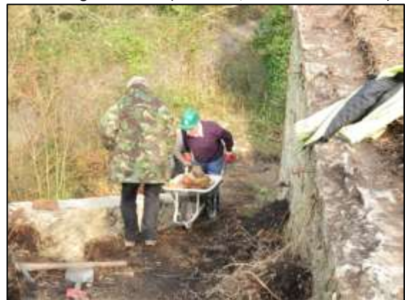
Photo 61 – Backfilling the trench along the base of the Old Pit heapstead wall with rubble in March.
