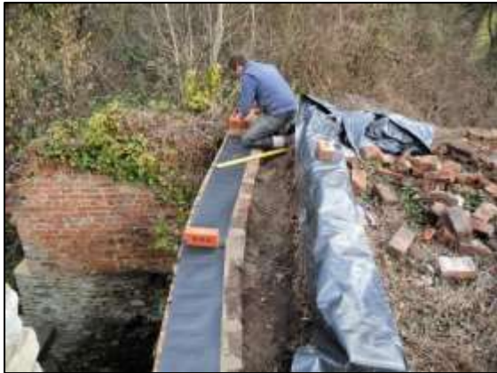
Photo 31 – ... a mason starting to lay the brick capping onto a damp proof membrane ...
