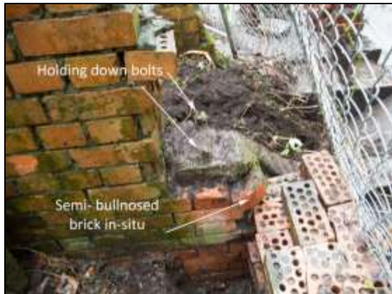
Photo 44 – The holding down bolts, located at the eastern end of the fan ducts, are thought to be part of the supports for the fan bearing.
