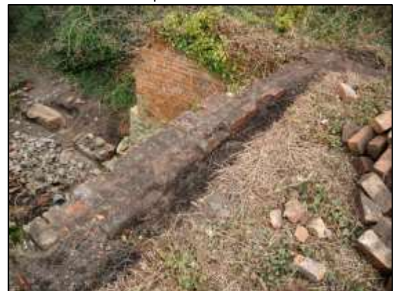
Photo 30 – A section of top of the wall of the Old Pit heapstead, located above the Old Boiler House, cleared of vegetation and ready for recapping ...
