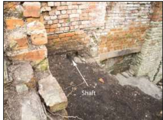
Photo 18 – View of the platform above the Pumping Shaft passage, after the flagstones had been removed during the rebuilding of the wall on the right of the photo. The position of the stone-lined shaft seen in the following photo has been marked.
