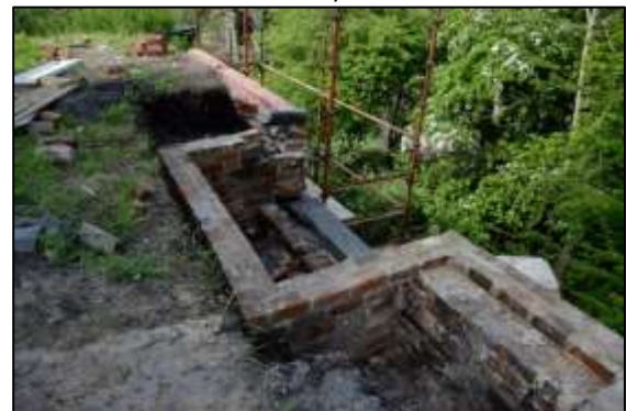
Photo 42 – The rebuilt southern tippler slot on 14 May.
