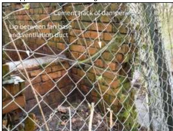
Photo 45 – The fan end of the northern duct, showing the cement track associated with the movement of the damper.
