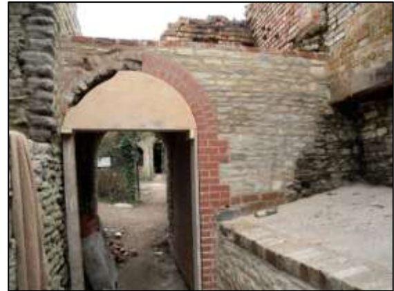
Photo 16 – Rebuilding of the wall above the Pumping Shaft and inside the adjacent passage in progress.
