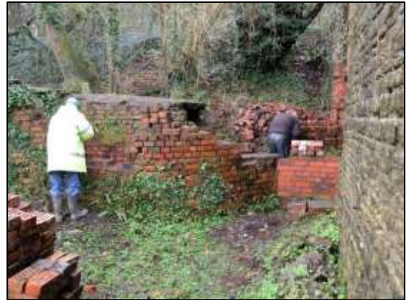
Photo 22 – Clearing around the fan ducts in January 2016 in preparation for the reconstruction of the duct walls.
