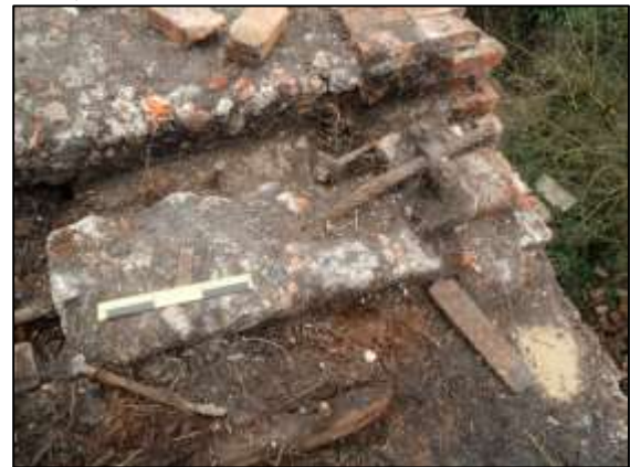
Photo 48 – The eastern rope has been bent back on itself and anchored in a block of concrete. The winding shaft lies out of view on the left of the photo. (30 cm scale)
