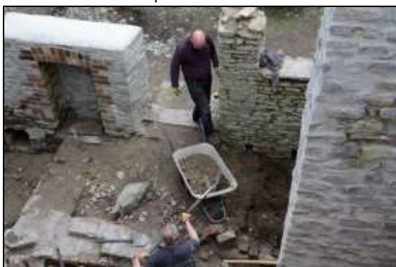
Photo 64 – Clearing the narrow trench between lines of holding down bolts in the Vertical Engine House in April. This probably housed the flywheel.
