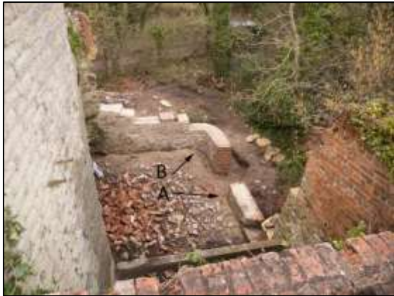
Photo 7 – The rebuilt north-western and north-eastern walls of the Old Boiler House in mid-March, seen from the Old Pit heapstead. The letters A marks the section of wall seen in photos 3 and 4, while B marks the section seen in 5 and 6.
