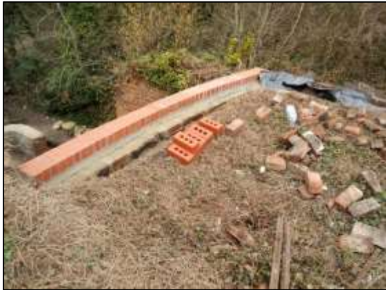
Photo 32 – ...and the completed capping in place.
