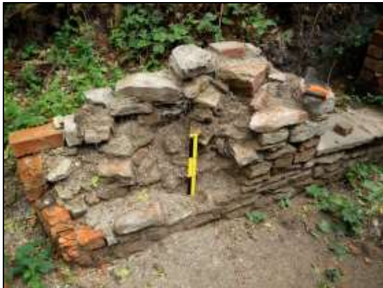
Photo 3 – Part of the north-east wall of the Old Boiler House in September 2014. The rebuilt section is marked as 'A' in photo 7. (30 cm scale)
