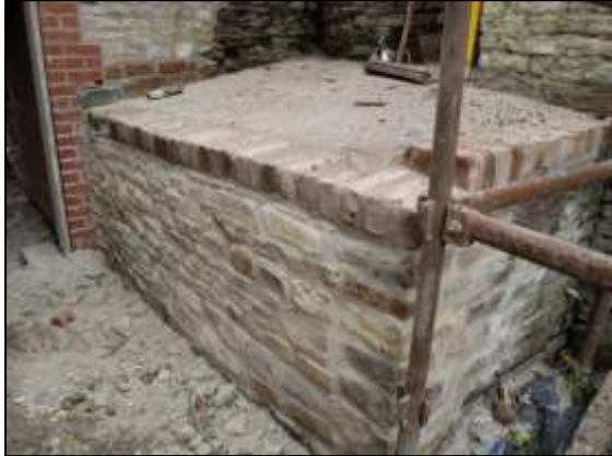
Photo 15 – The rebuilt base of the Pumping Shaft capping in March 2016.
