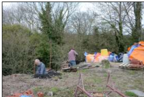
Photo 65 – Work in progress on the tippler slots of the Old Pit heapstead, with stockpiles of builder's supplies on the right of the photo.
