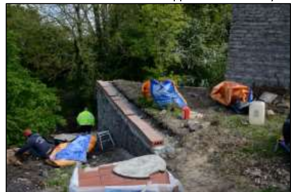
Photo 43 – The wall above the Old Pit heapstead ramp on 14 May after recapping was completed.
