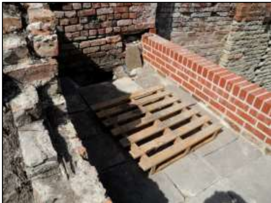
Photo 20 – The platform in May after the wall had been built up, and the flagstones re-laid. The area around the top of the shaft has still to be finished off and a grille installed.
