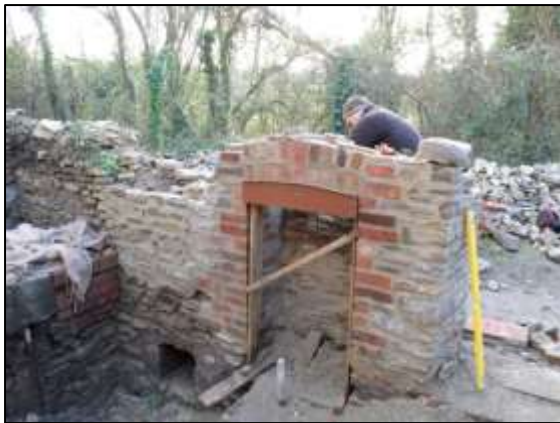
Photo 54 – The rebuilding of the south-east wall of the Vertical Engine House, and its inset fireplace, on 10 February 2016.
