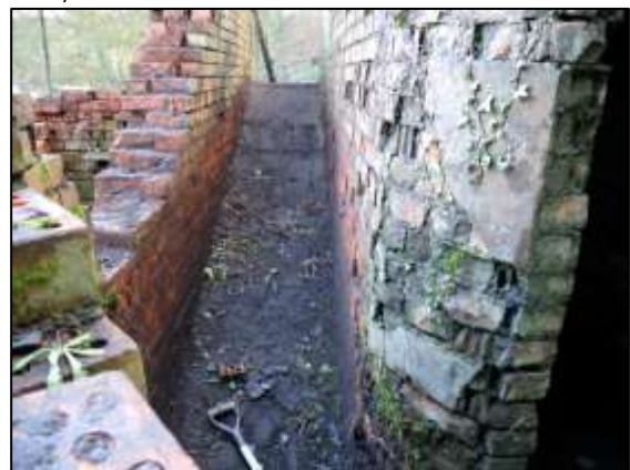
Photo 59 – The sloping floor of the northern fan duct, viewed from the heapstead end of the duct.
