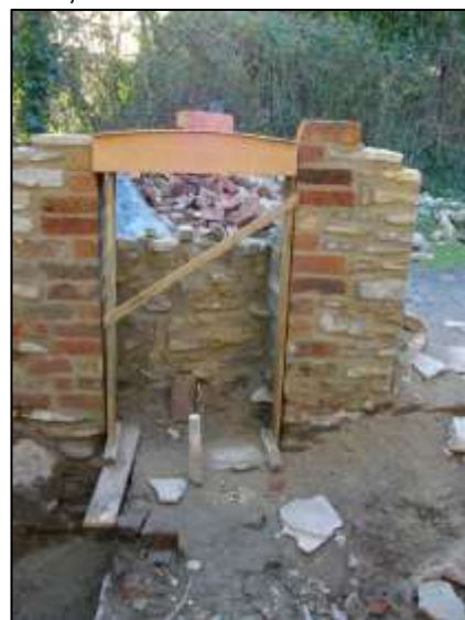
Photo 53 – A relatively early stage in the rebuilding of the south-east wall of the Vertical Engine House. (© K Kemp)
