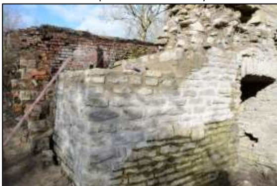
Photo 48 – A buttress is being built at the southern end of the bob (north-western) of the Cornish Engine House.
