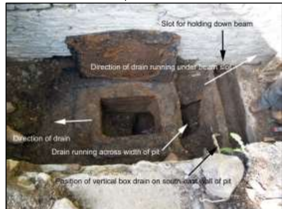
Photo 40 – Drain in base of winding drum pit, Vertical Engine House.
