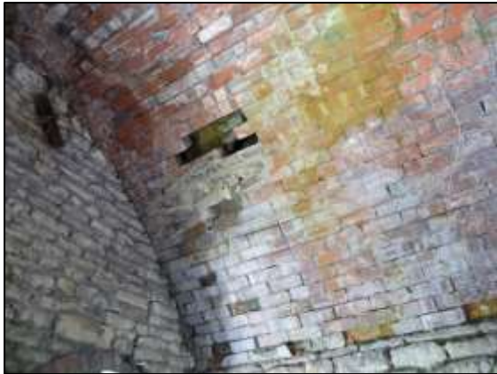
Photo 7 – Eastern corner of the inside of the Horizontal Engine House after most of the missing bricks had been replaced.
