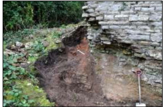
Photo 11 – Close-up of the eastern corner of the Cornish Engine House before rebuilding ... (1ft scale in centre of photo)
