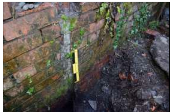
Photo 58 – The damper in photo X closed against this cement seat in the southern wall of the duct. (30 cm scale)
