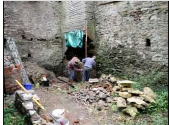
Photo 69 – An early stage in the rebuilding of the base of the chimney.
