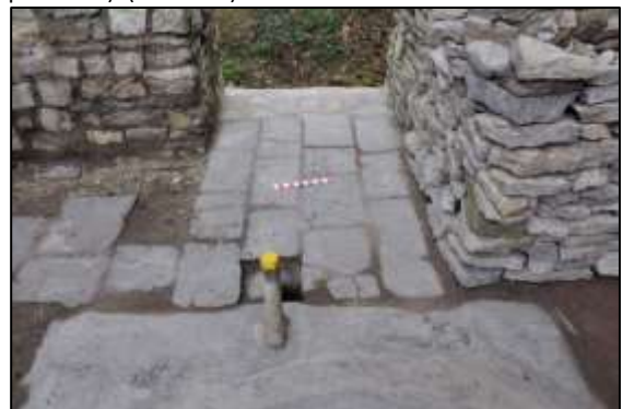
Photo 14 – Stone slabs covering part of the floor of the Cornish Engine House, with the engine bed in the
