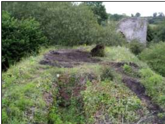
Photo 29 – A large hawthorn stump, and other vegetation, had to be removed from the roof of the Horizontal Engine House before the waterproof membrane could be laid...
