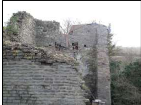
Photo 44 – Top of south-east wall of Cornish Engine House in background on 23 January 2016 after repairs to masonry of southern corner...
