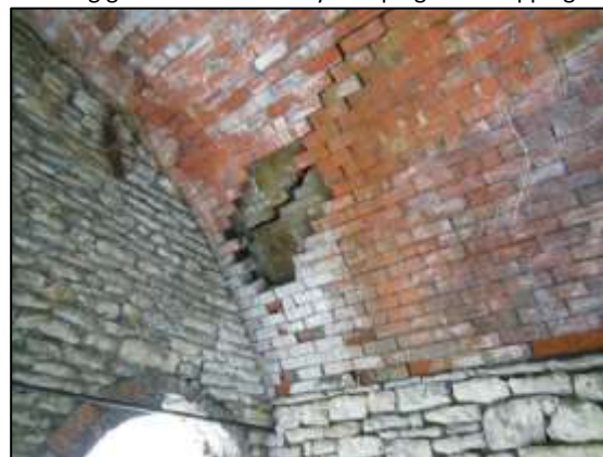
Photo 6 – Eastern corner of the inside of the Horizontal Engine House. The dark area in the middle of the photo shows the area where the outer layer of bricks had fallen. Running through that area is a crack in the next layer of bricks.
