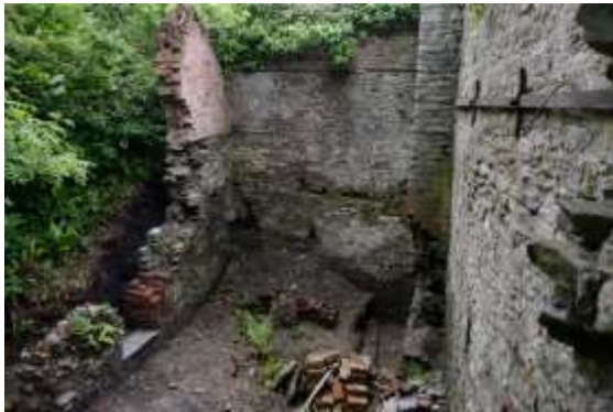
Photo 37 – The bulge in the north-east wall of the Old Boiler House can be seen in the left of the photo. This has been caused by pressure from material in the batch to its left.
