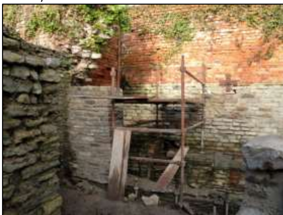
Photo 55 – Building of a buttress against the south-west wall of the Vertical Engine House in progress on 10 February 16.
