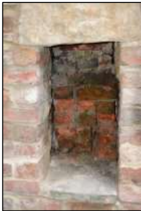
Photo 36 – Close-up of the rebuilt flue in the Old Boiler House.
