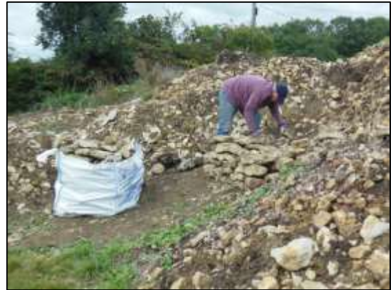
Photo 25 – Sorting out lias building stone from a dump.
