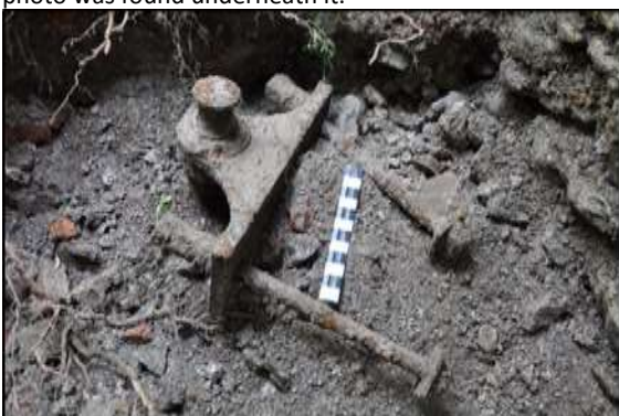
Photo 2 – Parallel motion bearing found in passage under the Pumping Shaft crossover. (1 ft scale)
