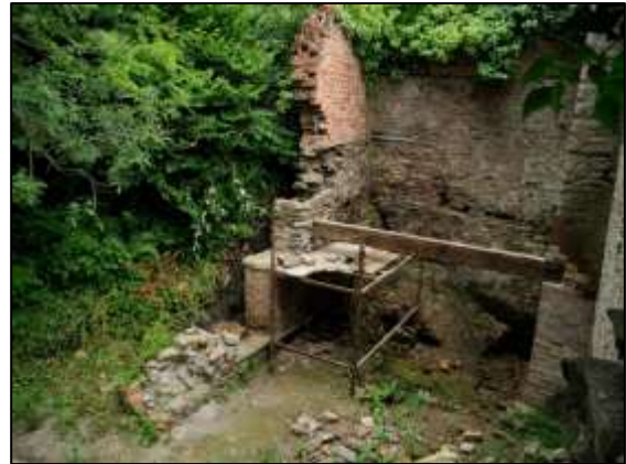
Photo 38 – Rebuilding of the north-east wall of the Old Boiler House in progress, with the bracing beam in place. The stone section of the wall has still to be built up to support the overhanging part of the brick section.
