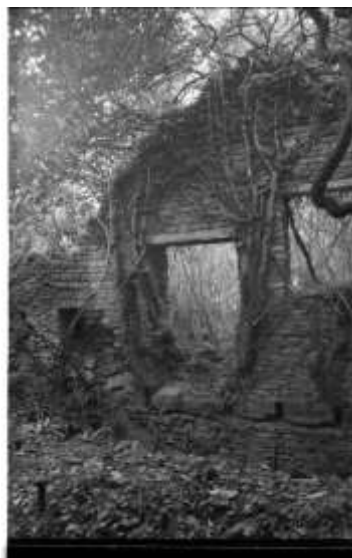
Photo 51 – The inside of the south-east wall of the Vertical Engine House in 1982. Note the fireplace to the left of the door opening in the centre. (@S Grudgings)
