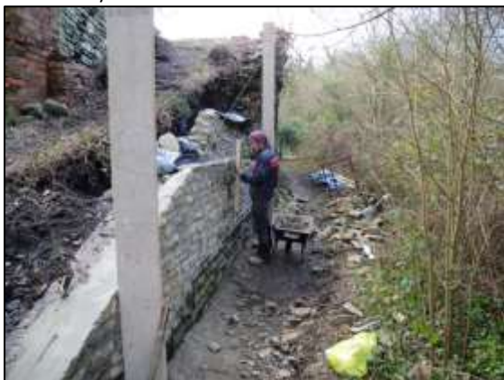
Photo 56 – Rebuilding the wall of the Old Pit heapstead ramp in progress on 10 February 2016.
