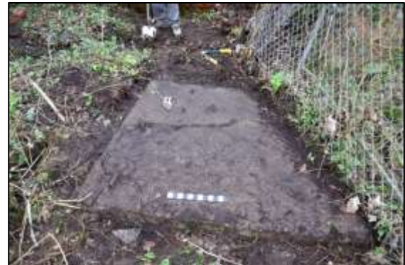
Photo 21 – Fan engine bed, with the fan ducts located just beyond the top right corner of photo. (1 ft scale)
