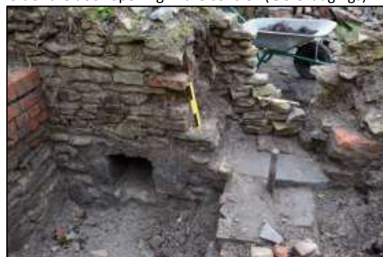
Photo 52 – Inside of south-east wall of Vertical Engine House before the rebuild started. The fireplace was located behind the remains of the holding down bolt, and the hole to its left is a channel through the wall. (30 cm scale)
