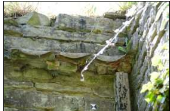
Photo 20 – Remains of roof tile fillets located on north-western wall of Horizontal Engine House.
