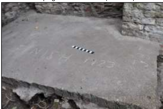
Photo 3 – Inscribed into the concrete of the Pumping Shaft capping is the phrase 'Finish 1923'. (1ft scale)
