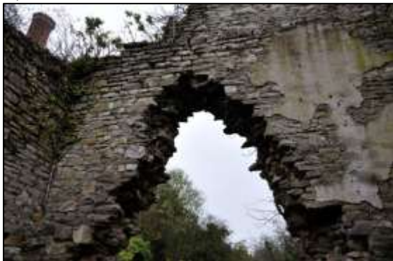
Photo 8 – The dogtooth gap of missing masonry in the north-east wall of the Cornish Engine House, taken from the inside of the building.
