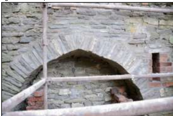
Photo 50 – ...and on 23 January 2016 after reinstatement of the arch and patching of the wall.
