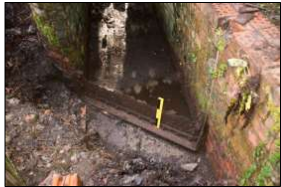
Photo 57 – Remains of a damper in the southern fan duct. (30 cm scale)
