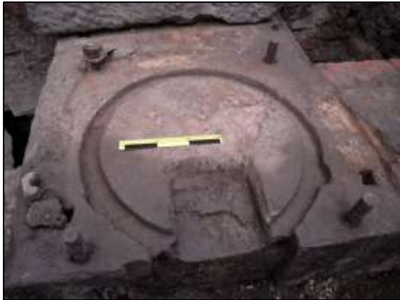
Photo 41 – A close-up of the engine bed in Vertical Engine House. Part of the cylinder casing is still attached to the bolt in the top left corner. (30 cm scale)
