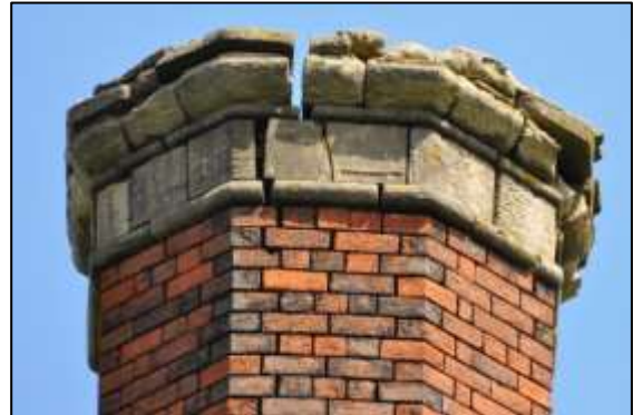
Photo 26 – The top of the chimney in 2011 showing the poor state of the stone capping, and the gaps between the stones where the cement had crumbled away. (This and photos 27 and 28 were all taken from approximately the same spot)
