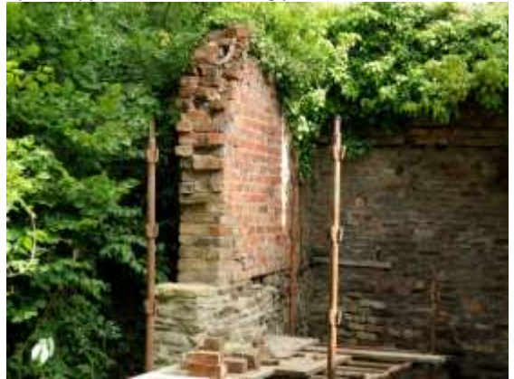
Photo 39 – Rebuilding of the north-east wall of the Old Boiler house almost complete.
