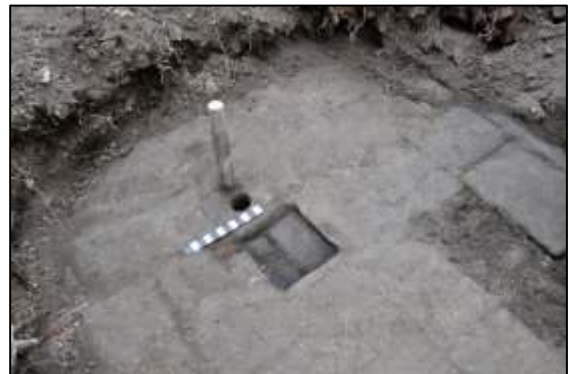
Photo 13 – North-eastern holding down bolt in Cornish Engine House with an empty socket beside it, seen from the north-east. (This feature has been reburied to protect it) (1 ft scale)
