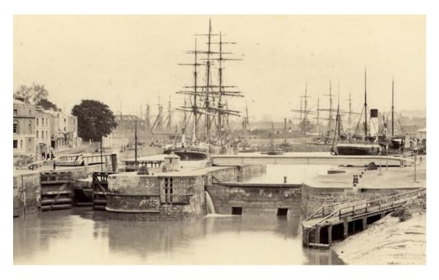
This amazing photograph shows Brunel's Lock on the right is closed by its floating caisson gate in which there are two square sluices. The present Swivel Bridge is in its original position over Brunel's Lock, and a copy is over Jessop's original north entrance lock.
