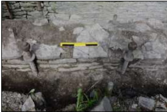
Photo 4 – Close-up of part of the central wall of the Vertical Engine House, with the winding drum pit in the background. (30 cm scale)
