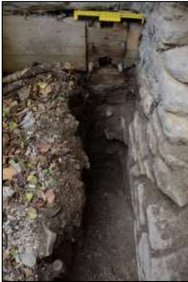
Photo 3 – Close-up of wooden plate (below 30 cm yellow/black scale) inset into the stonework of the south-western wall of the Vertical Engine House and fixed with 6 bolts.
