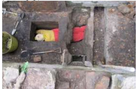
Photo 8 – Spoil being cleared from the drain under the winding drum pit. (© S Grudgings)
