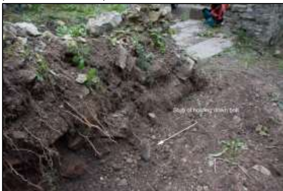
Photo 11 – Stub of holding down bolt next to the south-east wall of the Vertical Engine House, with the entrance door at the top right of the photo.
