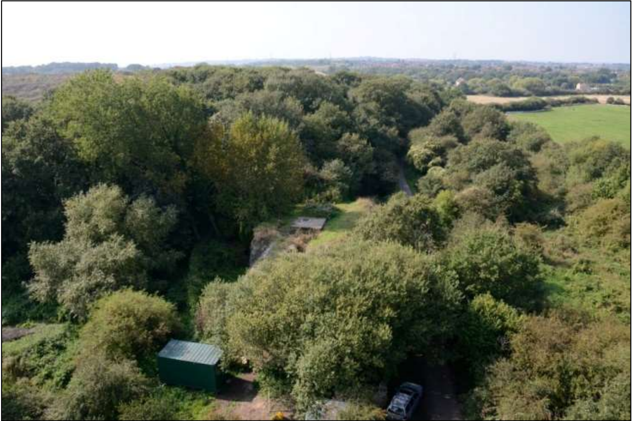
Photo 17 – View of the New Pit area from the top of the chimney. The container can be seen in the left foreground, with the Horizontal Engine House hidden behind the tree to its right. The pale-coloured square object in the middle is the New Pit shaft capping.
