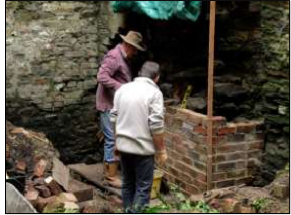
Photo 16 – Rebuilding the base of the chimney in the Old Boiler House.
