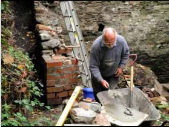
Photo 15 – Rebuilding the corner by the window in the Old Boiler House.
