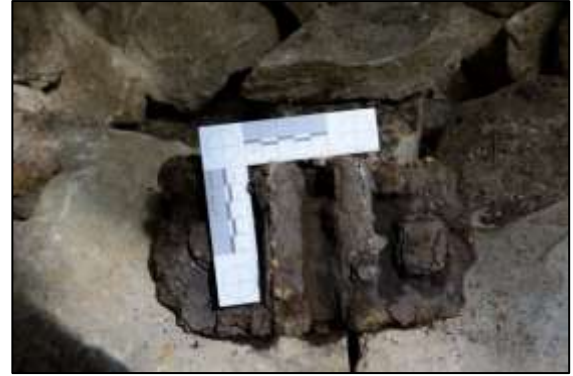
Photo 12 – Light rail chair found at base of north-west wall of the New Pit heapstead.
