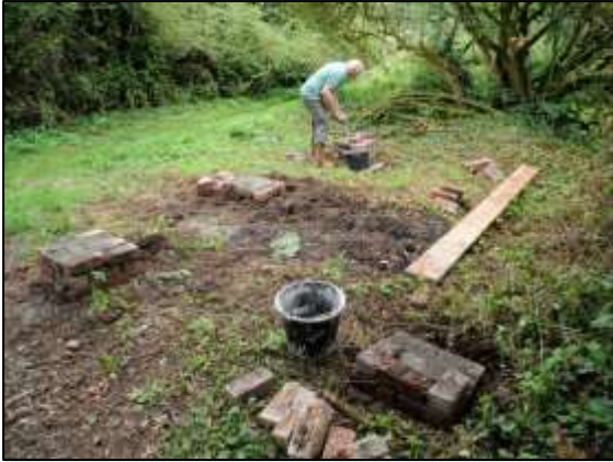
Photo 5 - Building the support pillars for the container.
