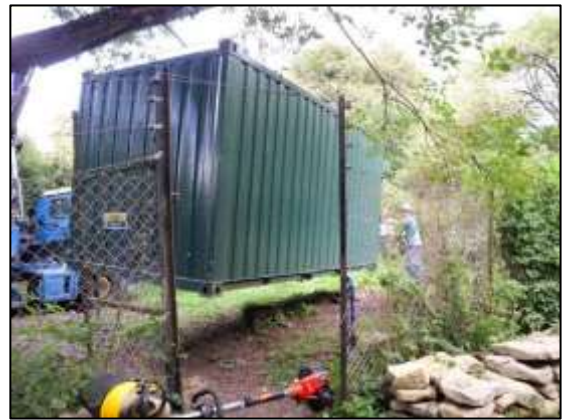
Photo 9 - Craning the storage container into position.
