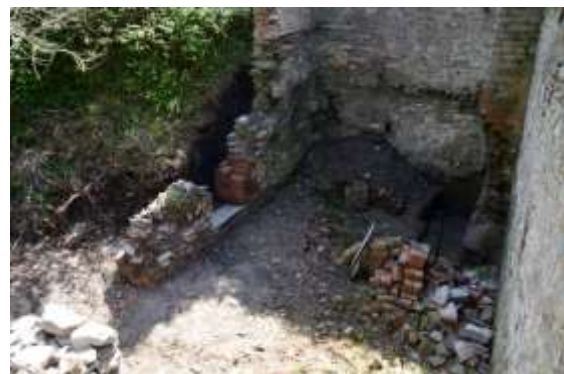
Figure 5 - Old Boiler House from heapstead ramp (03 May 14).
