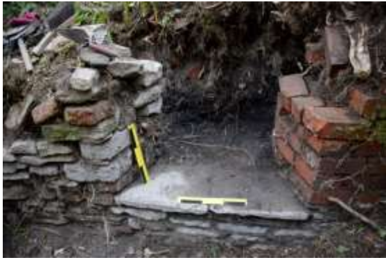
Figure 6 - Window opening in north-east wall of Old Boiler House.
