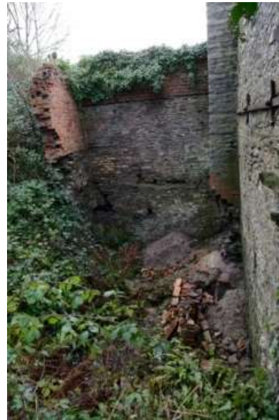
Figure 4 - Old Boiler House on 25 Jan 14 before clearance work started.
