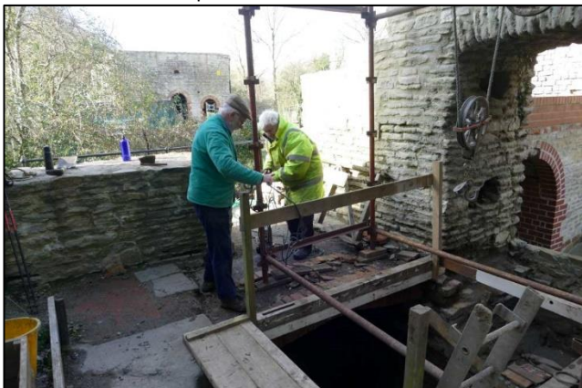
Photo 18 – Ken and Jeff setting up the pump used to dewater the bottom of the condenser pit.
