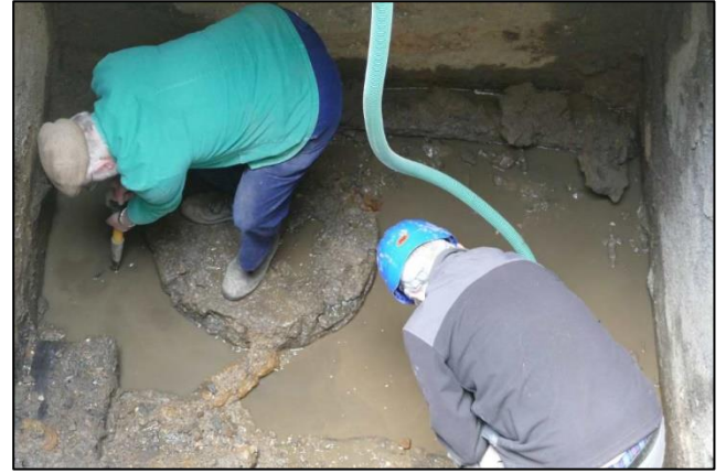
Photo 19 – Ken digs out sludge from the south-west end of the condenser pit, while Mark works the delivery line from the pump. The structure Ken is standing on can be seen more clearly in photo 15 opposite.
