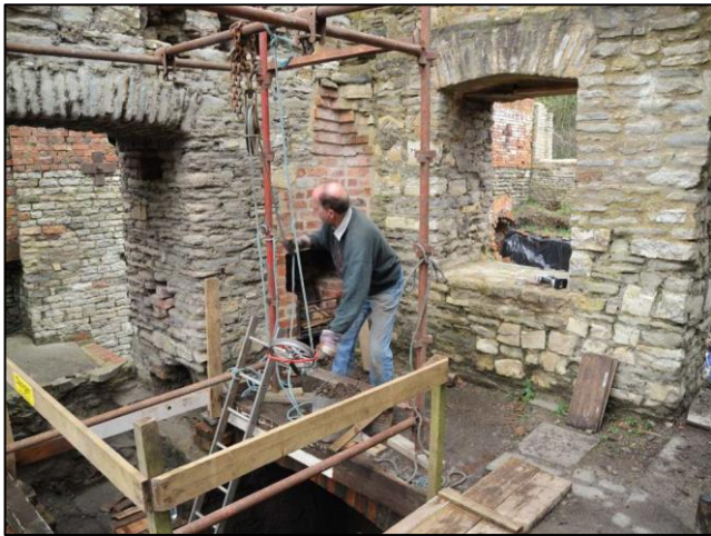
Photo 9 – Peter works the hoist located above the condenser pit of the Cornish Engine House ...
