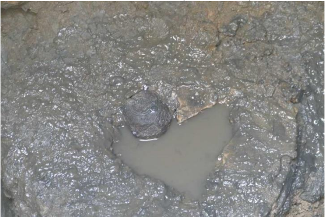
Photo 16 – Close-up of the wooden plug seen in the previous photo.
