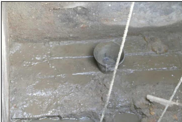
Photo 17 – Wooden planks embedded into floor of the north-east end of the condenser pit.
