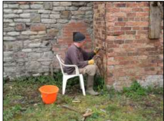
Photo 30 – Mick chases out the pointing at the south-west end of the Old Pit heapstead before fitting the stainless-steel ties.
