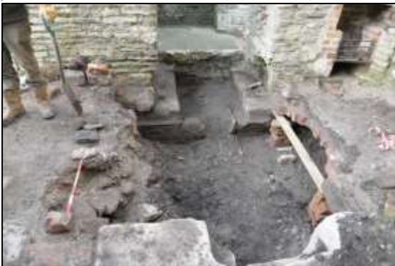
Photo 15 – View of the channel in the bob wall, seen from a position above the engine bed. Work has just started on excavating the roof of the south-west vault, seen on the left below the volunteer's boots.
