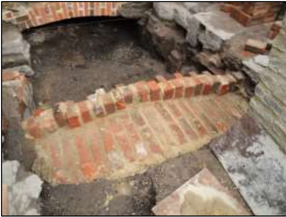
Photo 7 – ... and the completed first half of the arch.
