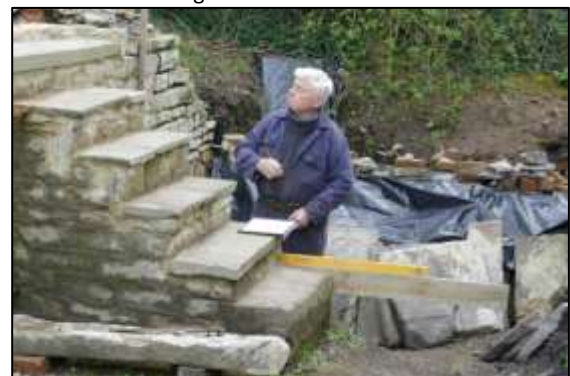
Photo 24 – Jeff studies the layout of the steps outside the Cornish Engine House as he takes the measurements he needs for making a set of handrails.
