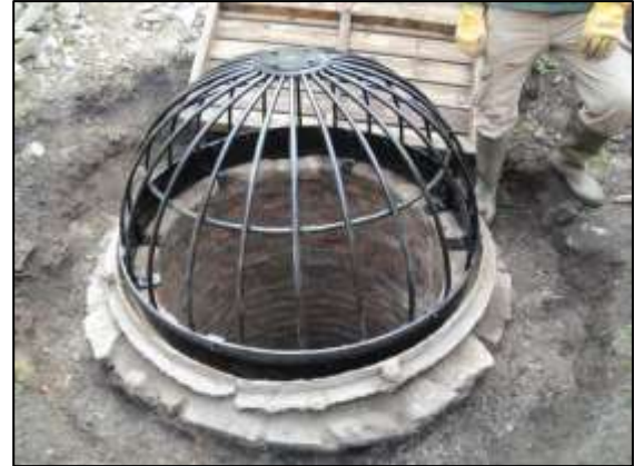
Photo 34 – Jeff has constructed a frame to cover the shaft.
