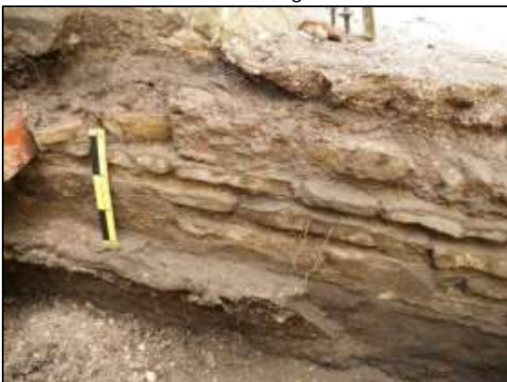
Photo 3 – This view of the inside of the south-west wall of the Cornish Engine House shows that the bricks of the arched roof of the vault on that side were not keyed into the masonry of the wall. (30 cm scale)
