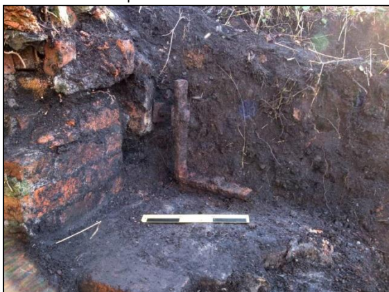
Photo 6 – Metal bracket in-situ in a slot at the top of the north-west wall of the New Pit heapstead. (30 cm scale)
