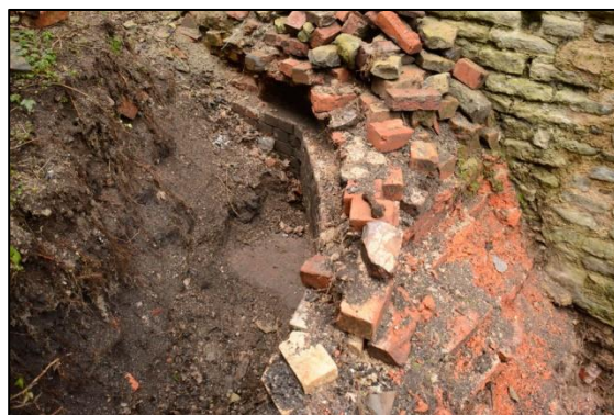
Photo 10 – Possible settings for the egg-ended boiler outside the eastern corner of the Cornish Engine House.
