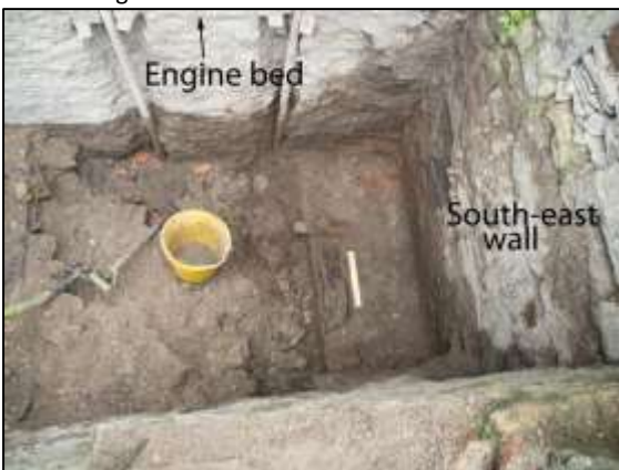
Photo 6 – Excavation of the pit below the engine bed in the Vertical Engine House has reached the level of the tops of the platforms. (30 cm scale)
