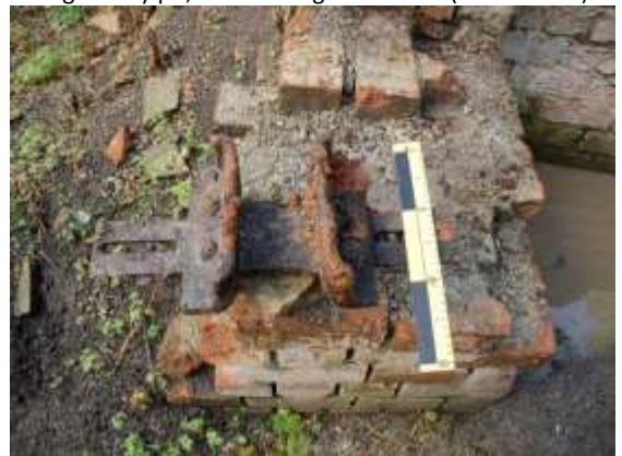
Photo 16 – Iron guide found in engine bay well, Vertical Engine House. (30 cm scale)
