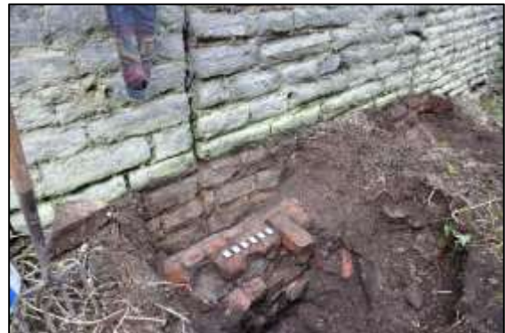
Photo 21 – One of the test pits dug outside the south-east wall of the Cornish Engine House in November 2012.
