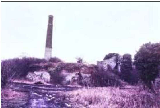
Photo 1 – Old Pit heapstead, with Cornish Engine House on the right. (© T Rendall, 1985)
