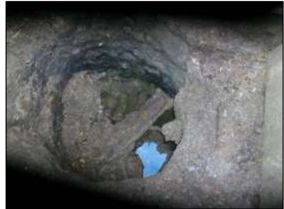
Photo 14 – Well in the engine bay pit, Vertical Engine House, at the start of a work party. (© K Kemp)
