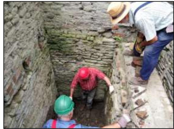
Photo 24 – ... and on 10 Aug when the excavation was much deeper.
