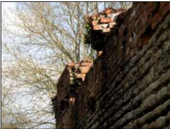
Photo 1 – North-west wall of Old pit heapstead from below, showing part of the brick pillar between the tippler slots balancing over the edge of the wall.
