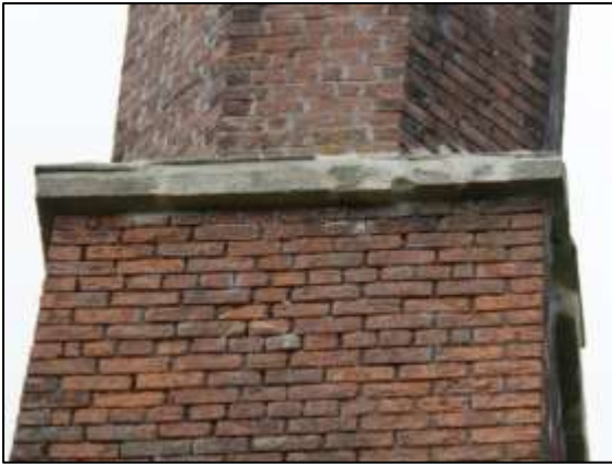
Photo 5 – ... and after the replacements had been pointed in.
