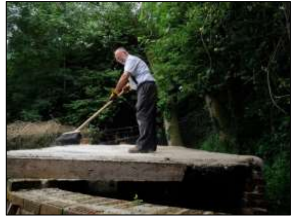
Photo 22 – Sweeping construction debris from the new roof of the Fan Ducts.
