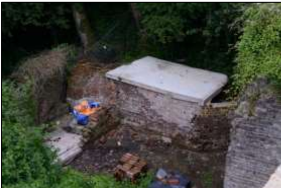
Photo 7 – Completed concrete roof over fan ducts in July 2016.
