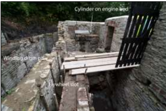
Photo 8 – View of Vertical Engine House from the south-west, with the positions of the engine bed, flywheel slot
