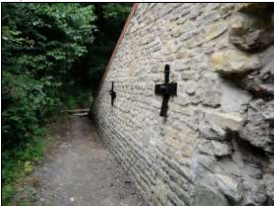
Photo 26 – ... and the finished result.
