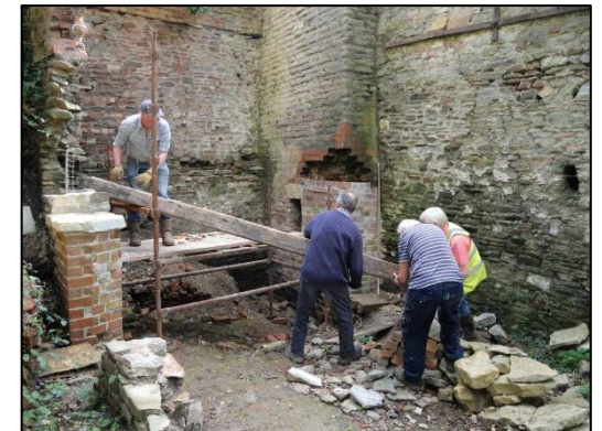
Volunteers installing a bracing beam in the Old Boiler House, April 2015.
