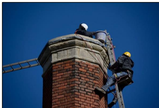
Contract masons working on the top of the chimney, February 2015.
