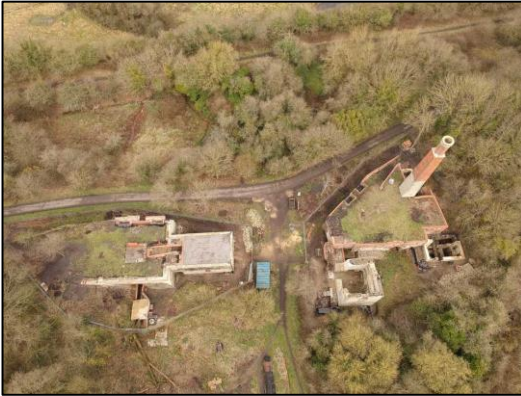
Aerial view of the site in April 2018, with the New Pit on the left and the original pit (Old Pit) on the right around the chimney. (Photo: © P Hodson)
