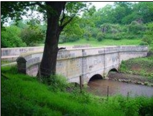
Downstream face of the restored Midford Aqueduct.
