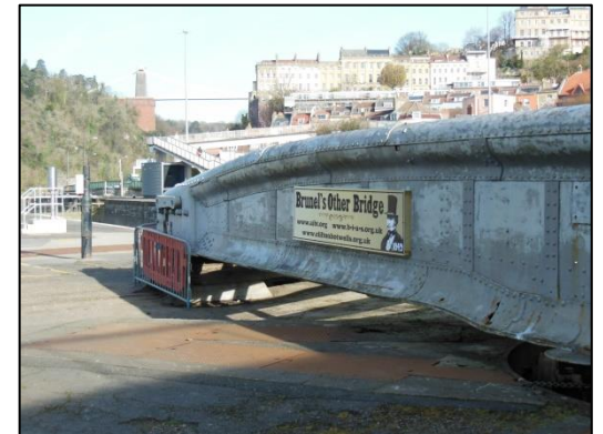
Brunel's Swing Bridge at the entrance to Bristol's Floating Harbour, with the Suspension Bridge in the background.
